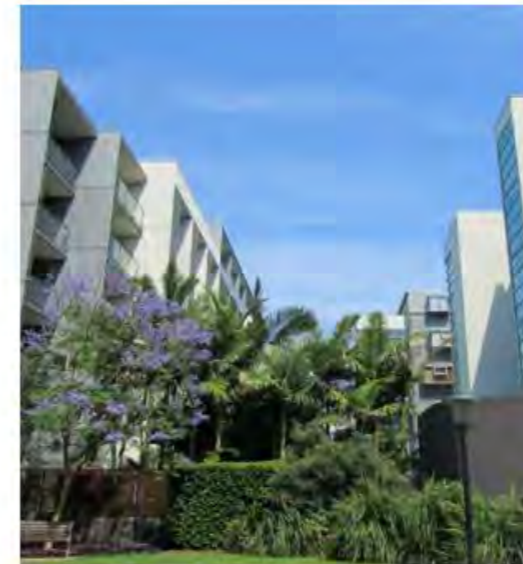
Figure 2F.3 Building separation supports residential amenity and helps to provide suitable communal open space areas
