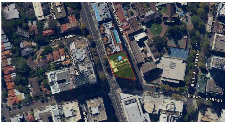
Figure 6: Aerial Image of the site, site highlighted in yellow (Source: Six Maps)
