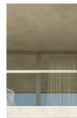
BL-02 GLASS BALUSTRADE Material: Frameless glass with flat aluminium top rail Finish: Clear
