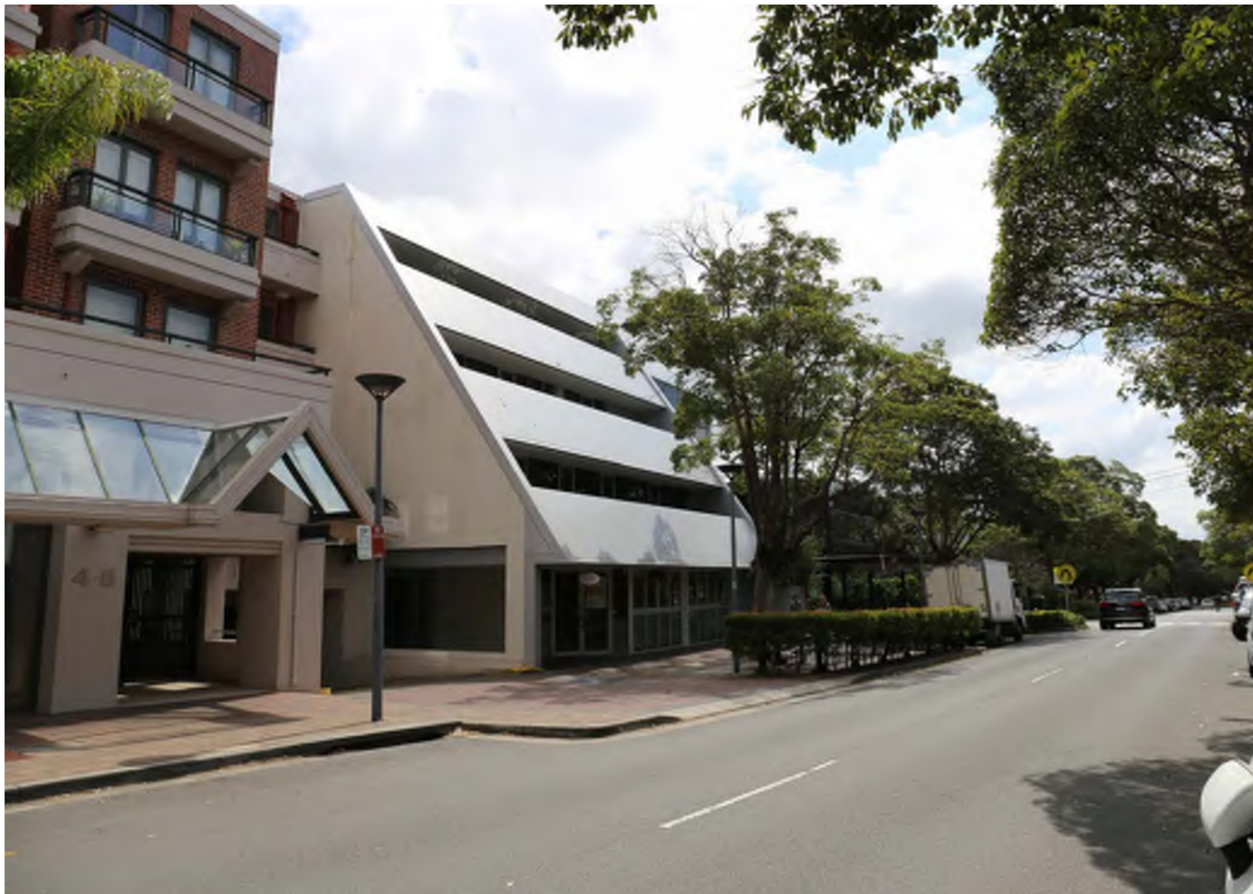
Image 1 - View looking North along Waters Road.
