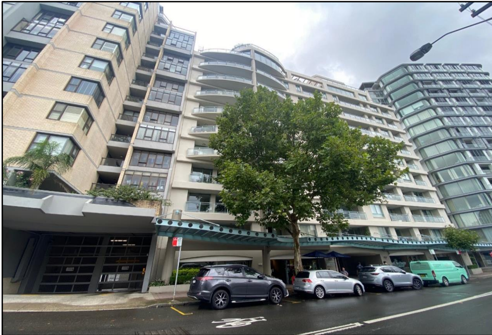
Figure 17 – Neighbouring building at No. 110-116 Alfred Street South
