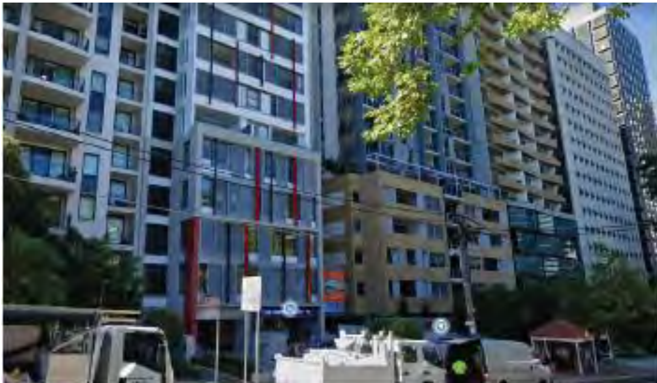
Figure 29 Recent Mixed-Use Tower Development along Miller Street
