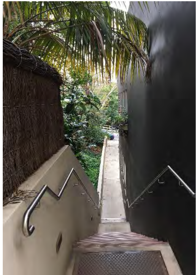
Picture 8: Existing through-site link, as viewed from Harnett Street
