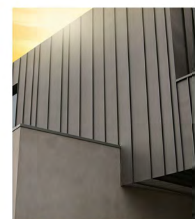
[2] TYPE: CLADDING MATERIAL: STEEL COLOUR: BASALT
