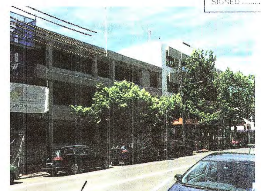
PHOTO EXISTING DEVELOPMENT ALEXANDER ST
