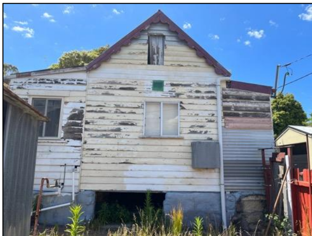
Photo 4: Existing western façade
