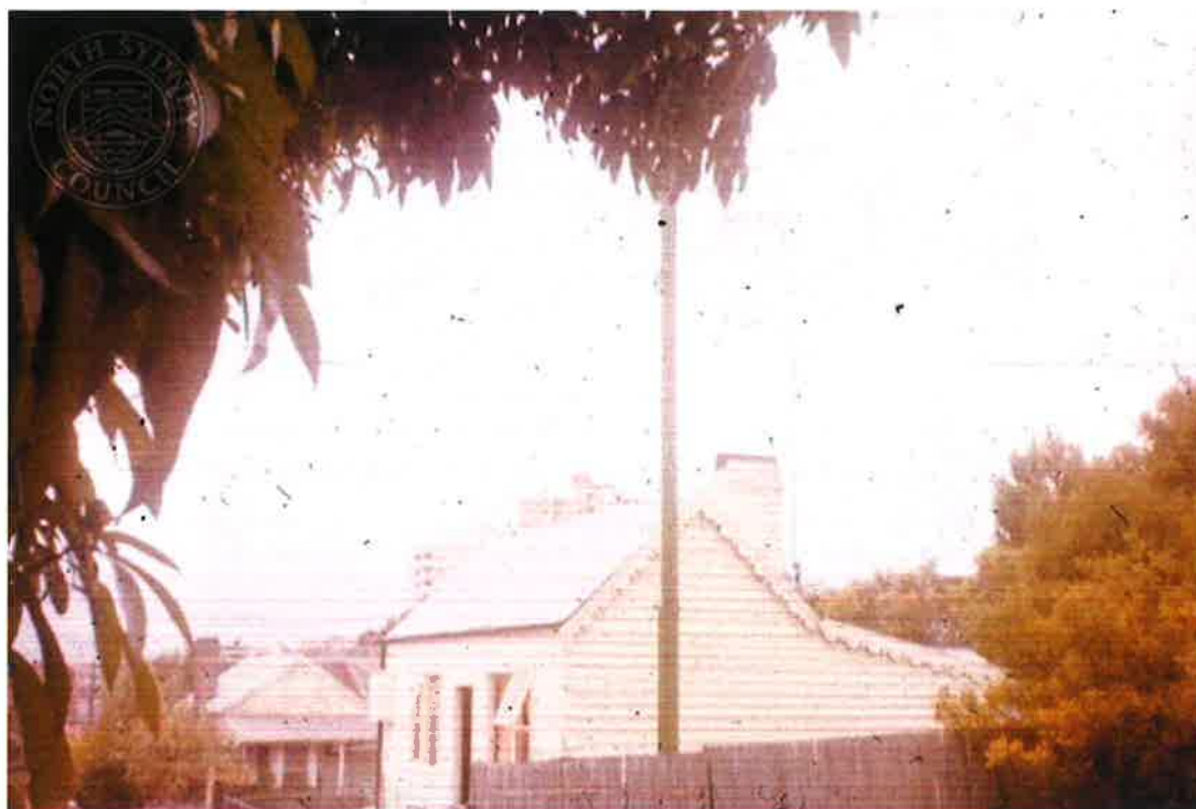
Figure 8: The house at 1 Bank Lane, 20 January 1976. Note that in 1976 the eastern extension to the cottage did not exist and there was no front verandah. Note decorative barge boards to eastern elevation in the foreground. Source: image courtesy Stanton Library
