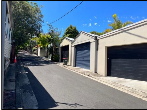
Photo 13: Existing garages on opposite side of Bank Lane
