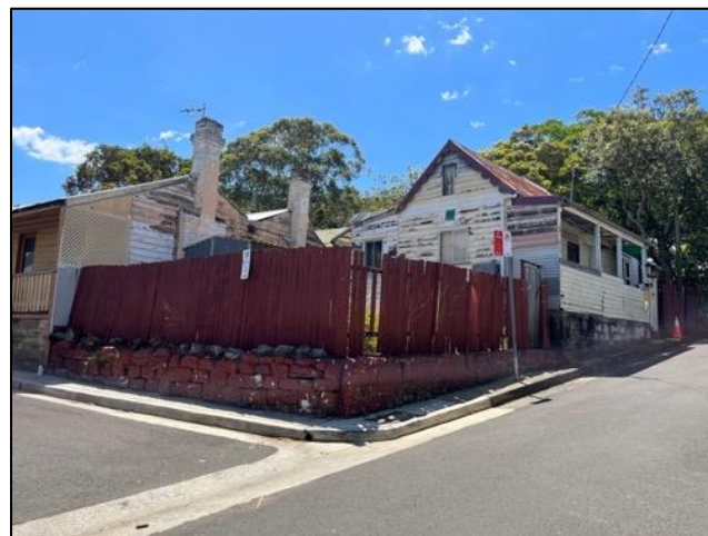
Photo 1: Existing dwelling viewed from corner of Bank Lane and Ancrum Street
