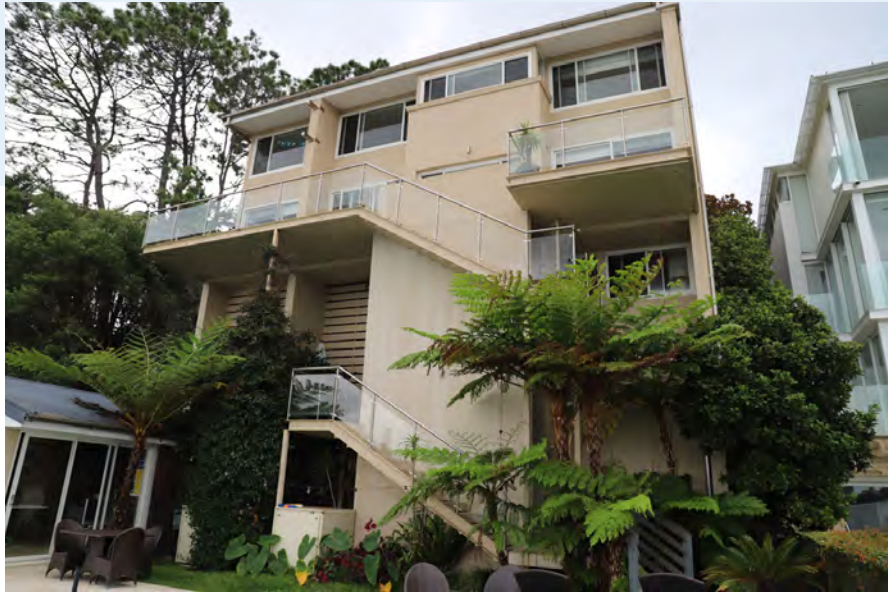
Photo. 12 Detail of the south elevation at 1 Baden Road
