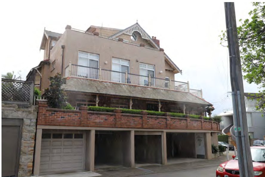
Photo. 14 Detail view of the south elevation at 2 Baden Road
