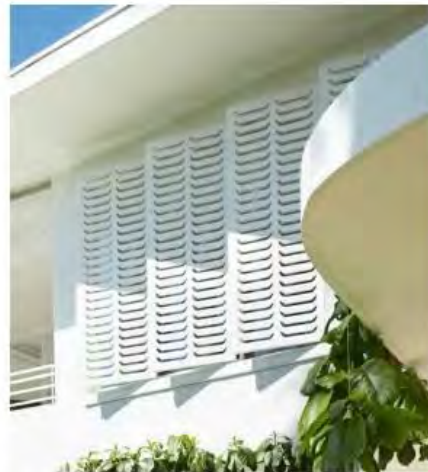
Figure. Proposed semi operable external timber shutters.
