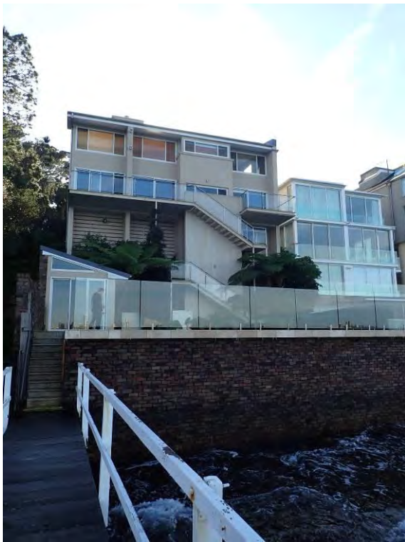
Figure 9. Site Photo of existing dwelling from the jetty
