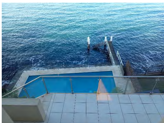
Figure 13. Site Photo of existing foreshore area
