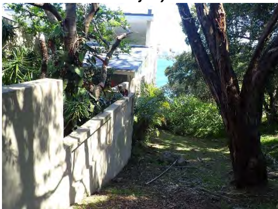
Figure 11. Site Photo of existing dwelling from Baden Road
