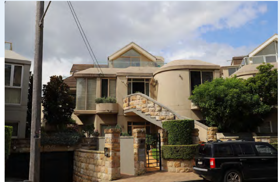
Photo. 22 Detail view of 9 Baden Road
