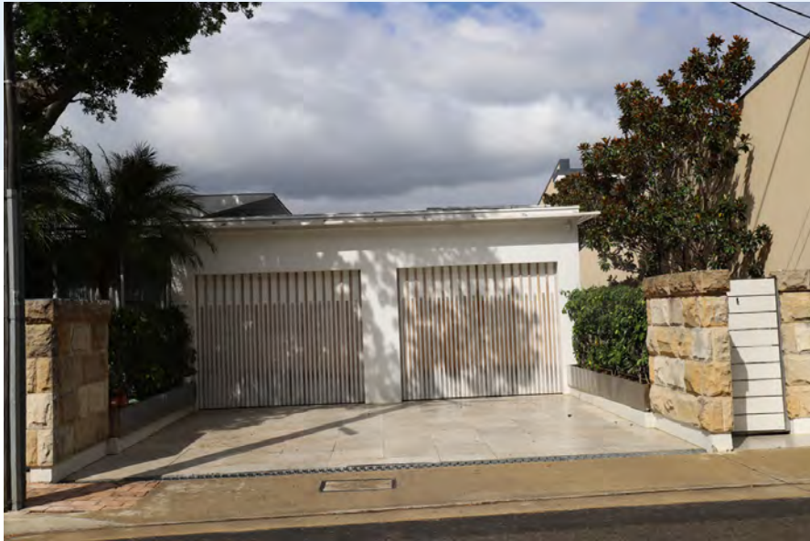
Photo. 18 Detail of 3-3a Baden Road Garage
