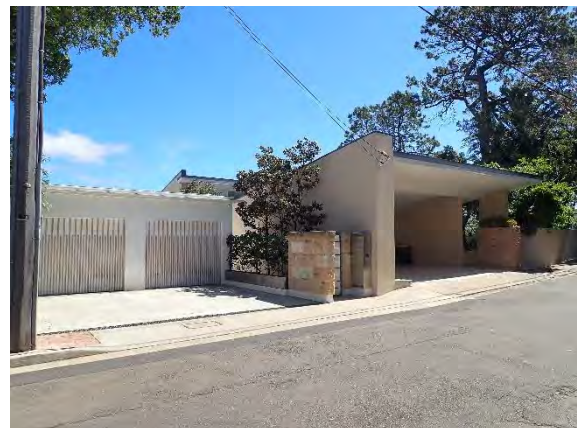
Figure 12. Site Photo of existing dwelling from Baden Road
