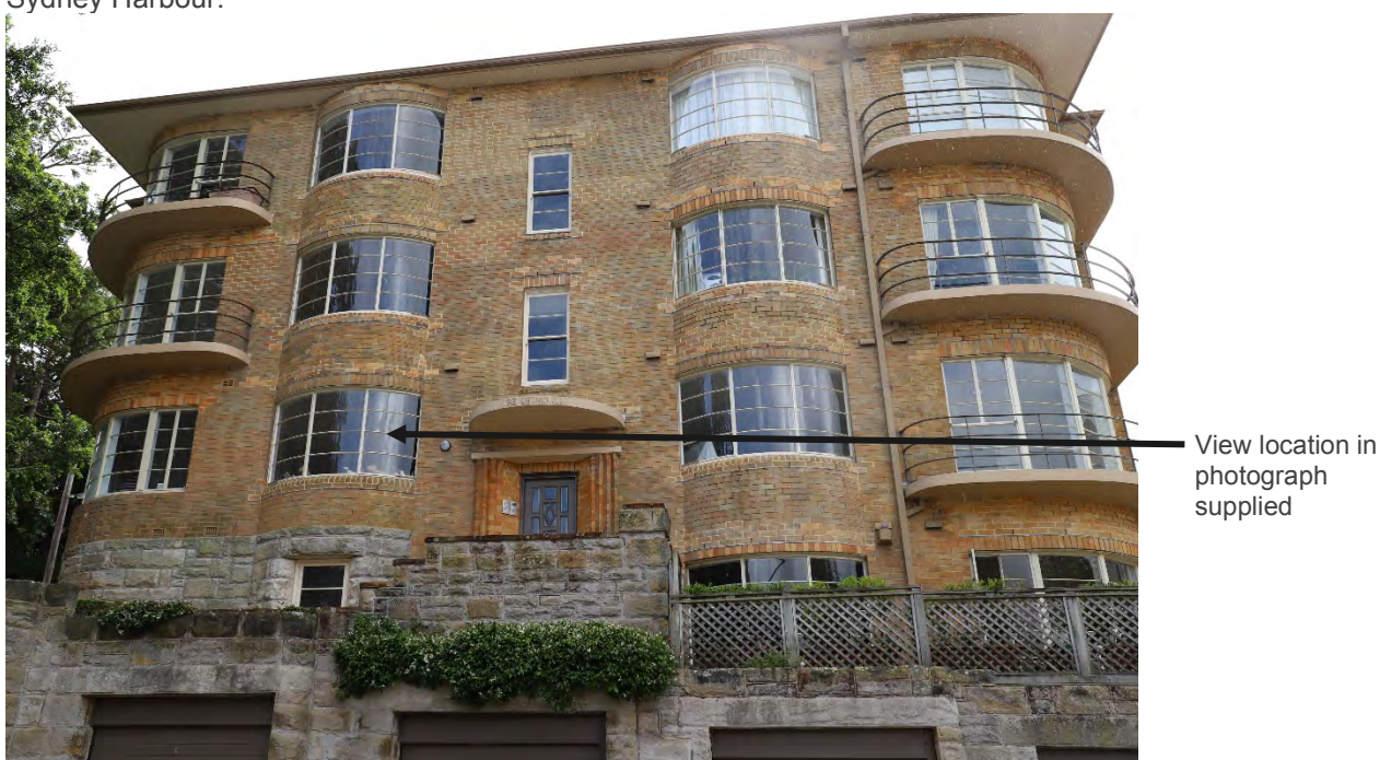
Figure 1 Detail of southern elevation of 200 Baden Road
