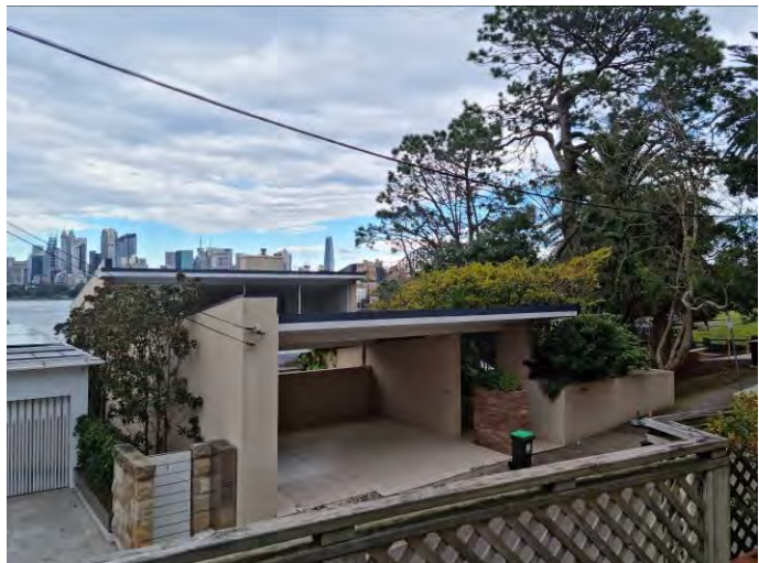
Figure 31. Site photo from southeastern corner of the front courtyard of Unit 7 No. 200 Kurraba Road.
