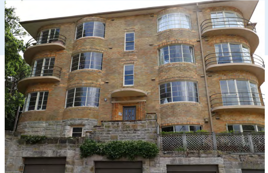
Photo. 16 Detail of the south elevation at 200 Kurraba Road showing the symmetrical layout of windows etc.
