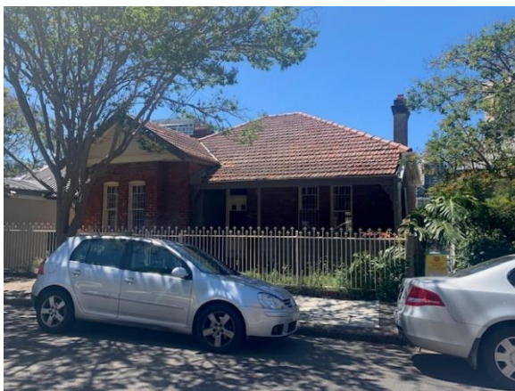
Image 4: 37 Bay View Street (adjoining)
