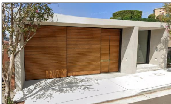
Photograph 5: No 3 Bay View Street with solid timber garage door
