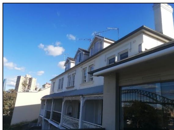
Photograph 3: Dormer windows at Nos. 27, 29 and 31 Bay View Street, as viewed from the upper-level terrace of the existing dwelling
