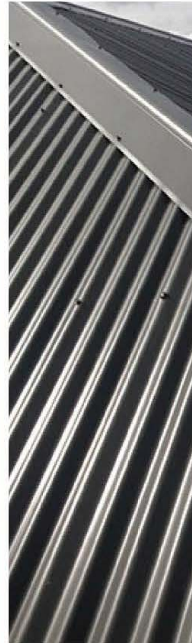
EXISTING ROOF SHEETING
