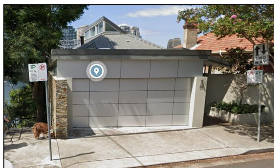
Photograph 6: No 39 Bay View Street with solid timber garage door
