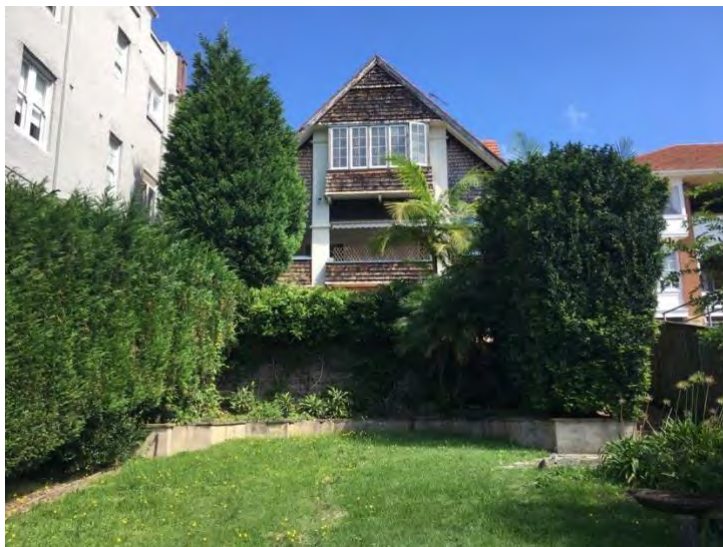
Photo 3 – View of existing rear/Eastern Elevation
