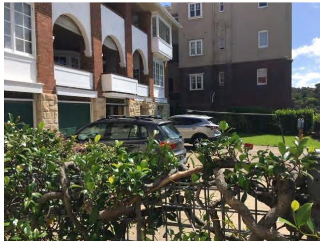
Photo 8 – Rear of No. 15 Shellcove Road
