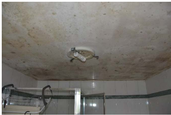
Figure 5.4.28: Plasterboard ceiling to Lower ground bathroom
