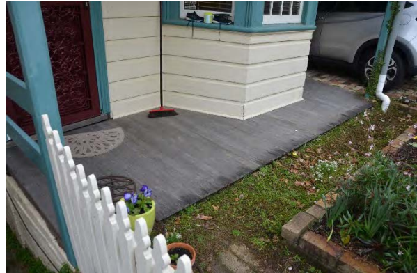
Figure 5.4.4: Front porch of neighboring 28 Thomas Street retains hardwood timber decking.
