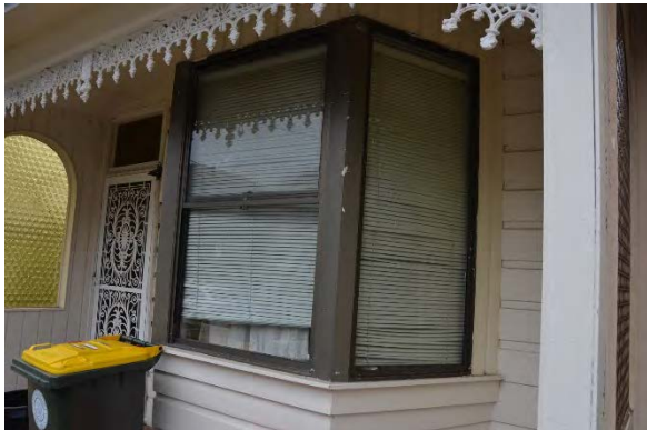
Figure 5.4.1: Front bay window addressing Thomas Street replaced with aluminum. Front elevation consists of modern weatherboards (replacing original splayed weatherboard).
