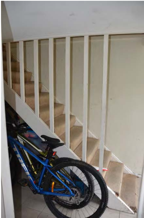
Figure 5.4.25: Stair to lower ground level added in 1981.
