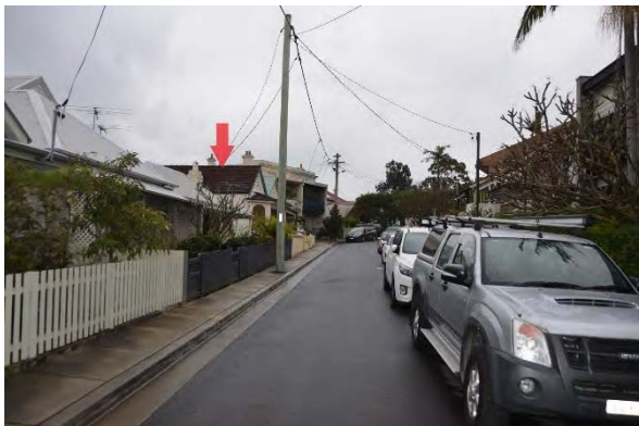
Figure 5.2.3: View looking northwest along Thomas Street with 26 Thomas Street visible on the left (marked by an arrow).
