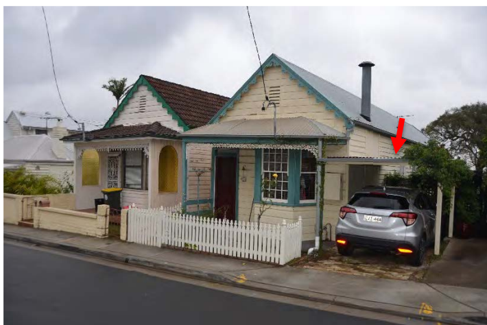
Figure 7.4.5: Existing view of the 26 and 28 Thomas Street from a similar angle showing the low-profile carport for 28 Thomas Street.
