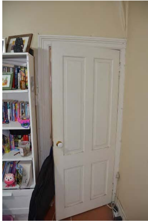
Figure 5.4.17: Second room. Original architraves with replica four panel door.
