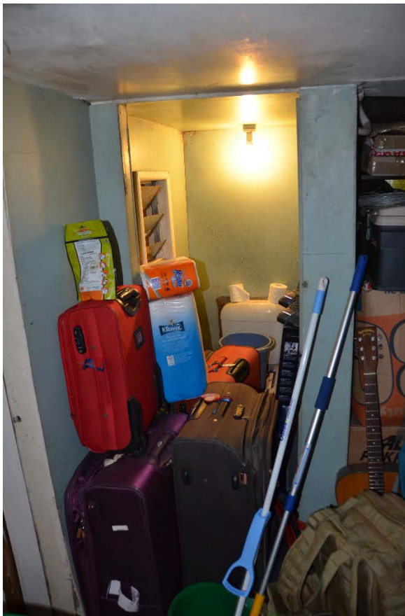
Figure 5.4.31: Late 20 th Century toilet room in the laundry area.
