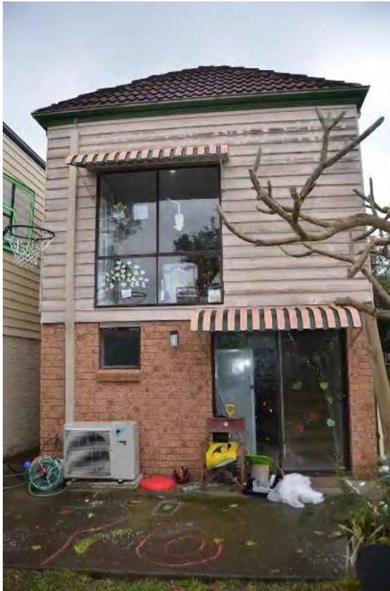
Figure 5.4.6: Rear elevation consisting of brick lower ground floor and shipped lapped weatherboard first floor and aluminum windows.
