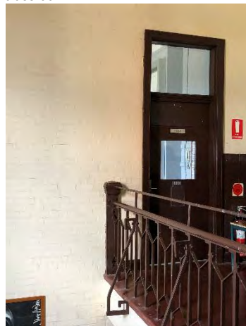
Figure 23: Balustrade with additional top railing
