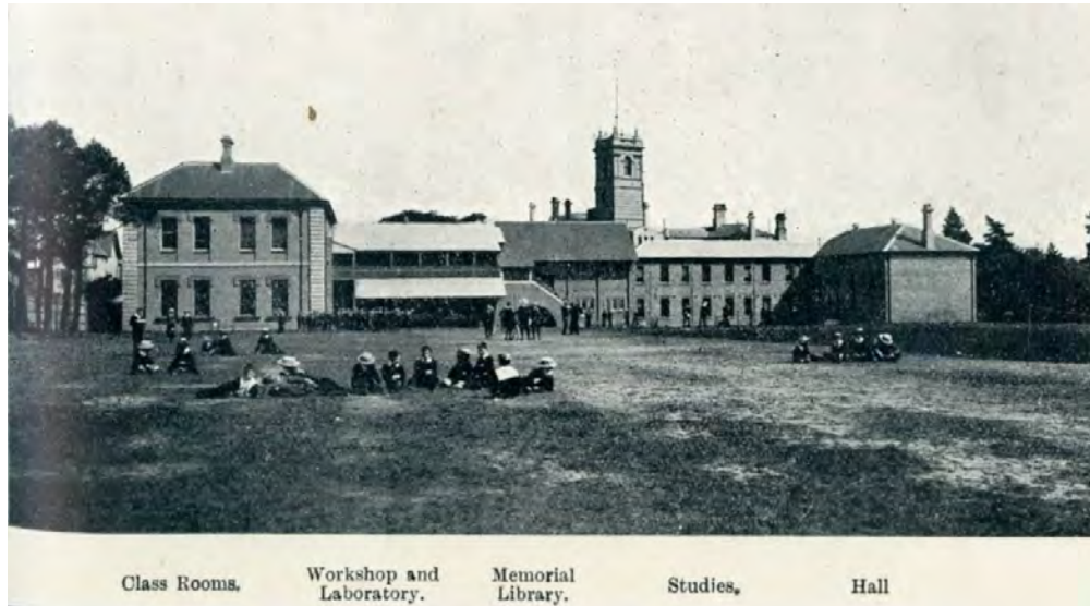
Figure 7 – Northern elevation of Shore showing from left to right original two-storey classroom block (Building 13), workshop and laboratory, memorial library, boarders studies and hall (now building 14) - pre-1920. (Source: Shore Archives, west_742)
