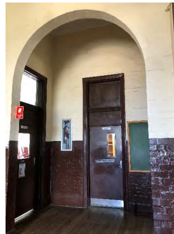
Figure 24: Entry to office to east of stairwell
