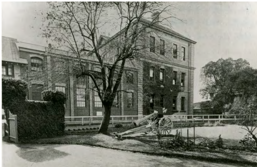
Figure 8 – The classroom block and laboratories, about 1922 after the additional floor was erected. (Source: Shore Archives, BC19/20)
