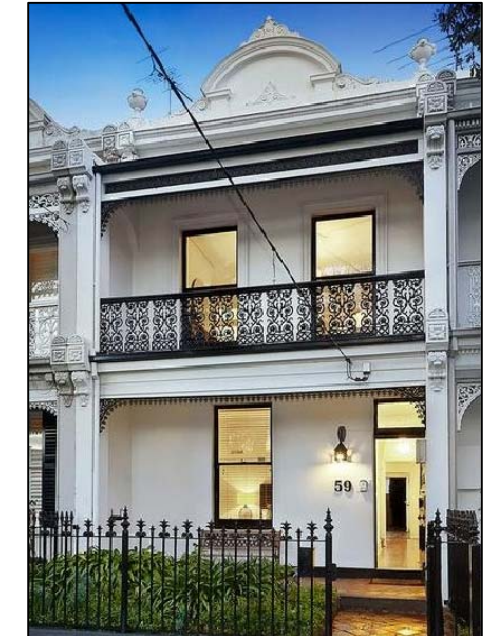
ORNAMENTED PARAPETS & PROJECTING VERANDAH WING WALLS ⑦
