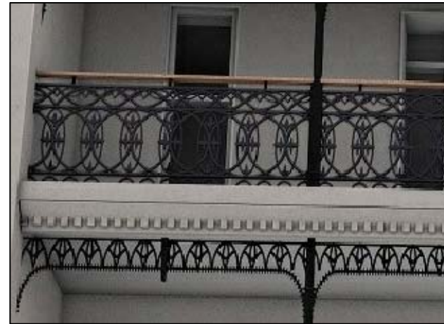
CAST IRON BALUSTRADES - DULUX COLORBOND MONUMENT ⑤
