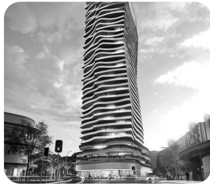
3. THE LANDMARK (UNDER CONSTRUCTION) 44-STORY TOWER+EQUALLY TALL TOWERS ARE BEING CONSTRUCTED IN THE CENTRE+STATION
