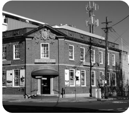
7. FORMER BANK PROMINENT STREETSCAPE ITEM+INTERWAR REVIVAL OF GEORGIAN ARCHITECTURE (ITEM NO. 10151)
