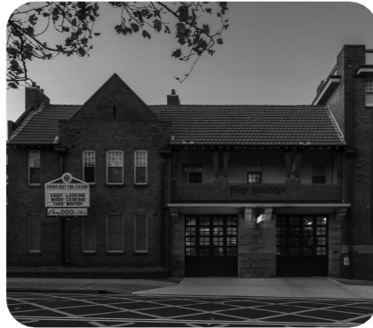
9. CROWS NEST FIRE STATION ARTS+CRAFTS STYLE IN PUBLIC UTILITY; ONE OF LAST STATIONS DESIGNED BY GOVERNMENT ARCHITECT (ITEM NO. 10173)
