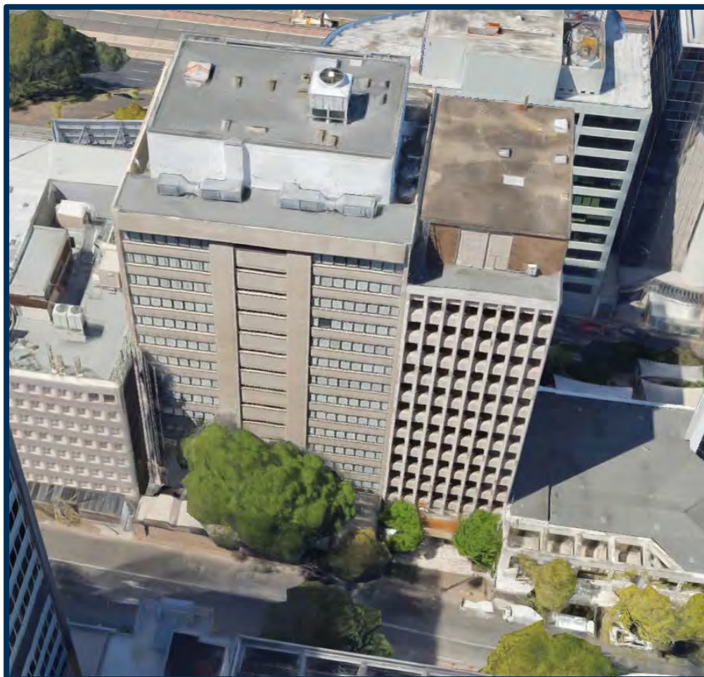
Figure 8 View of the existing commercial office buildings occupying the site
