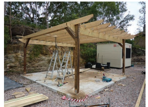
Caption: Construction of the potting shed shelter, May 2011.
