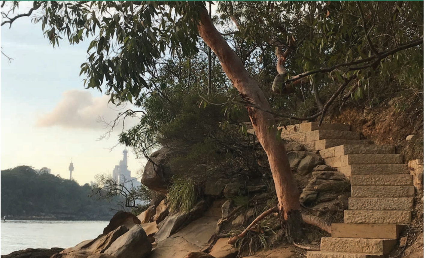
Caption: Sandstone staircase upgrade on the eastern Berry Island foreshore by Gareth Debney, 31 January 2020
