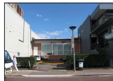
Rear of Military Road commercial building providing non-active frontage to Grosvenor Lane Car Park
