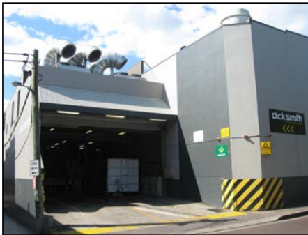
Supermarket loading dock in Grosvenor Lane
