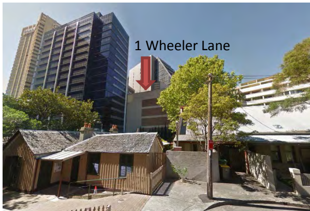
1 Wheeler Lane as viewed from Oak Street.
