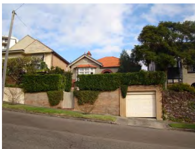
Figure B-13.28: Parking spaces combined with high fencing alienates the streetscape and is intrusive.
