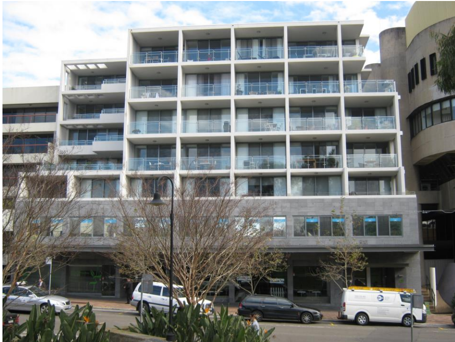
Figure 12 – Mixed use development at 26 Clarke Street
