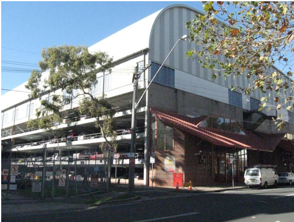
Figure 8 – Hume Street car park and North Sydney Indoor Sports Centre
