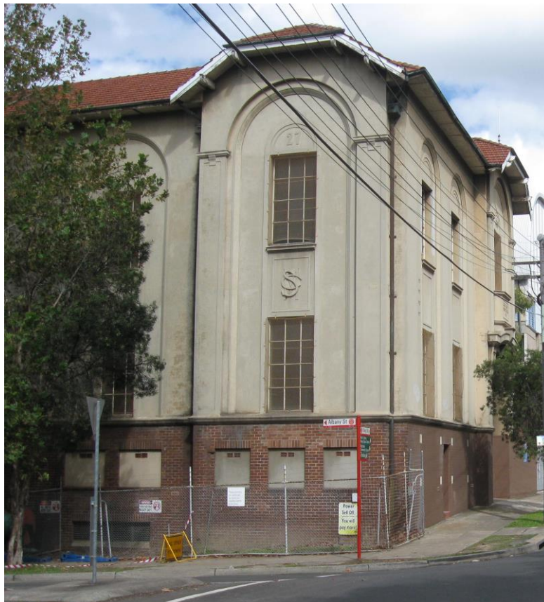
Figure 14 – The heritage listed electricity sub-station
