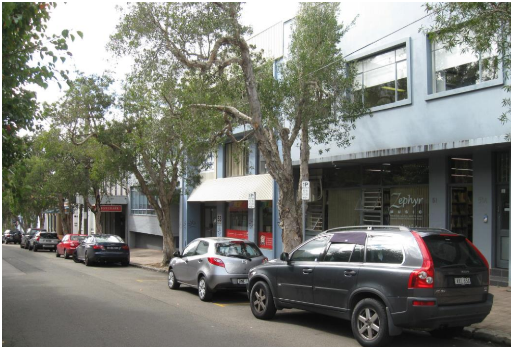
Figure 11 – Aging 2-3 commercial buildings on Hume Street
