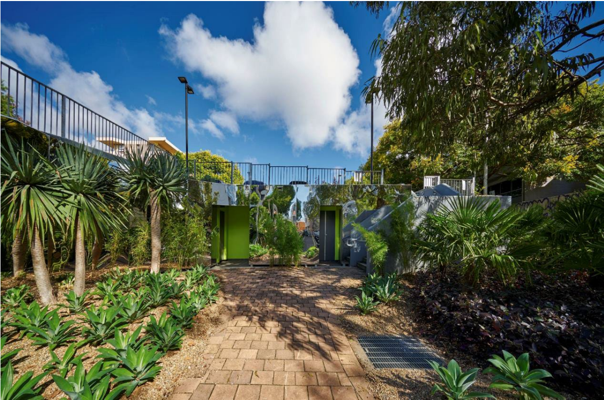
New Public Toilets have been built in the Barry Street Carpark – Neutral Bay in 2016 – costs $450K
