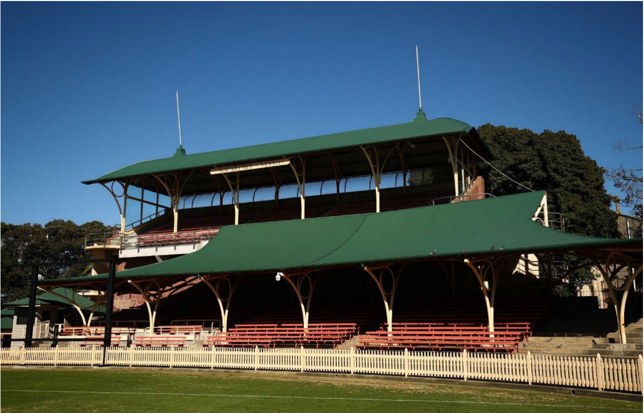
Councils Property team organise and undertake significant maintenance works on North Sydney Oval including roof replacement of the grandstands- painting and structural repairs each year.
