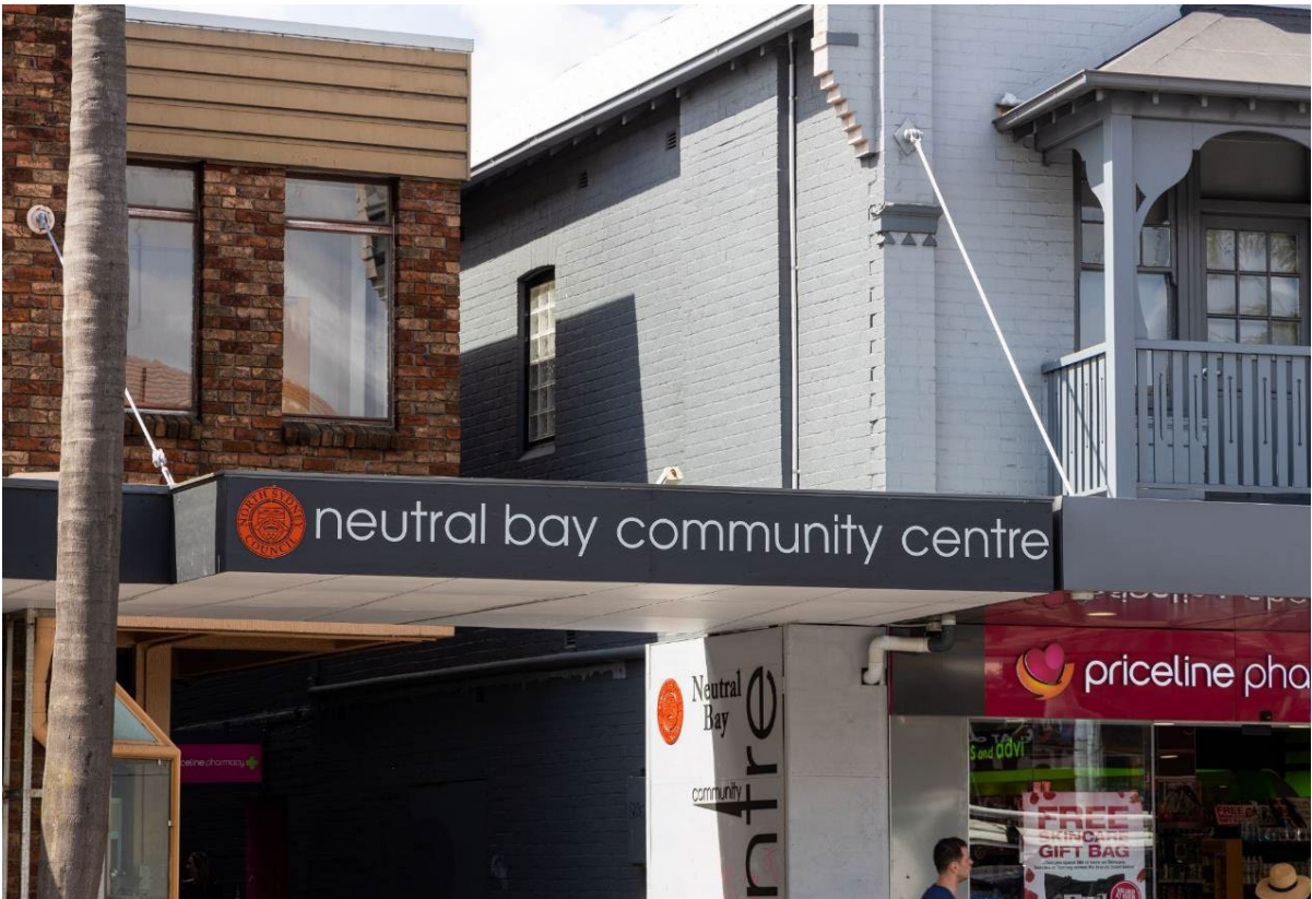
Upgrade of the Neutral Bay Community Centre – completed April 2019
