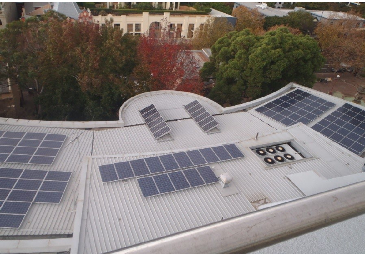
Solar Panels have been rolled out across a number of Councils Community and operational buildings over the last 5 years as part of an ongoing program. Stanton Library
