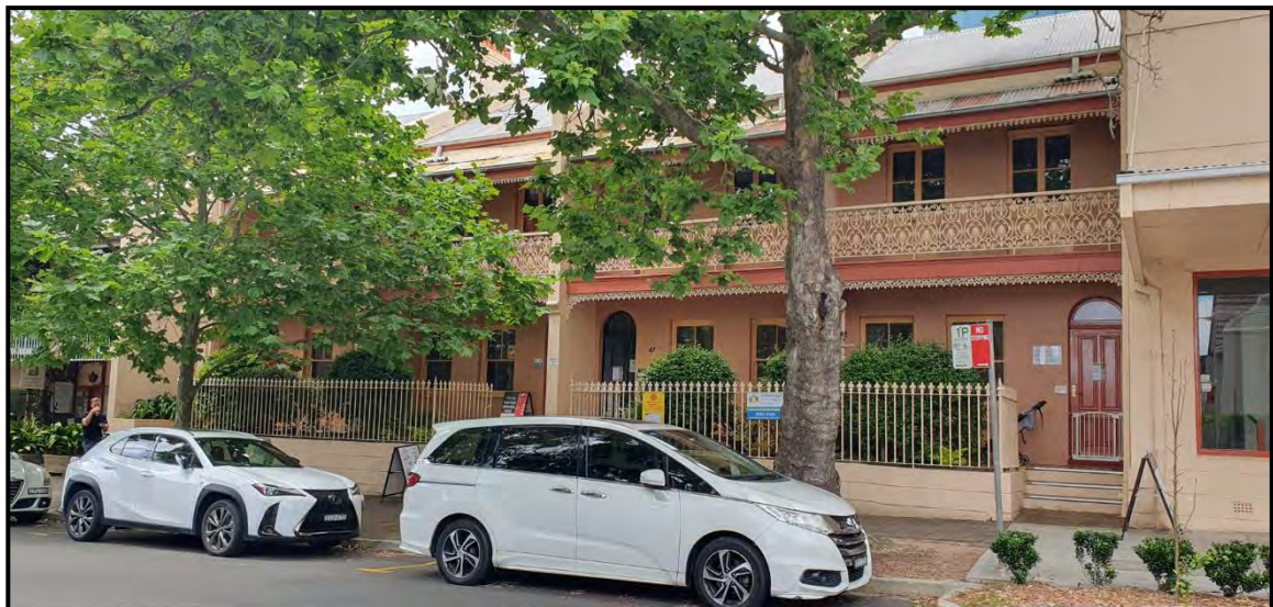
Figure 2: Ridge Street elevation, no alterations are proposed for the front (street/heritage) façade
