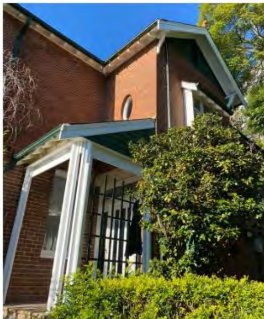
Figure 12. Principal entry west elevation
