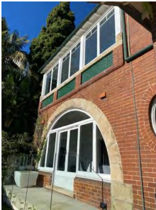
Figure 9. Principal front northern elevation
