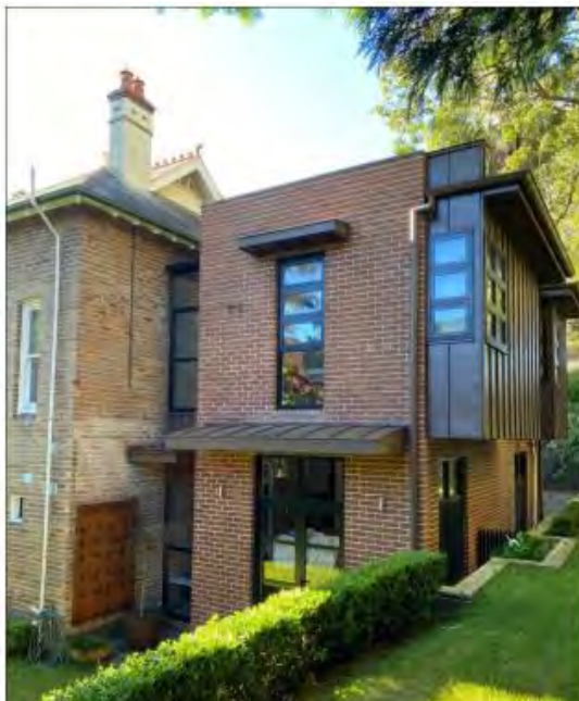
Figure 11. West elevation glass link at rear
