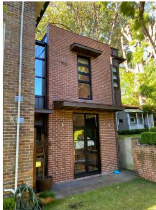
Figure 10. Western elevation rear addition
