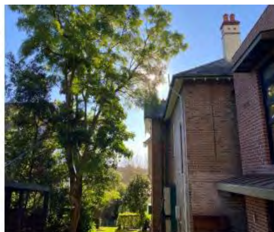
Figure 14. View north showing western elevation and roof profile
