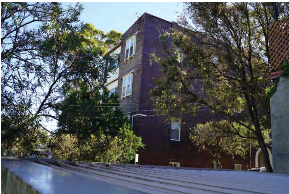
Plate 9 Haxton Court as viewed from the front yard of the subject site adjacent to the garage
