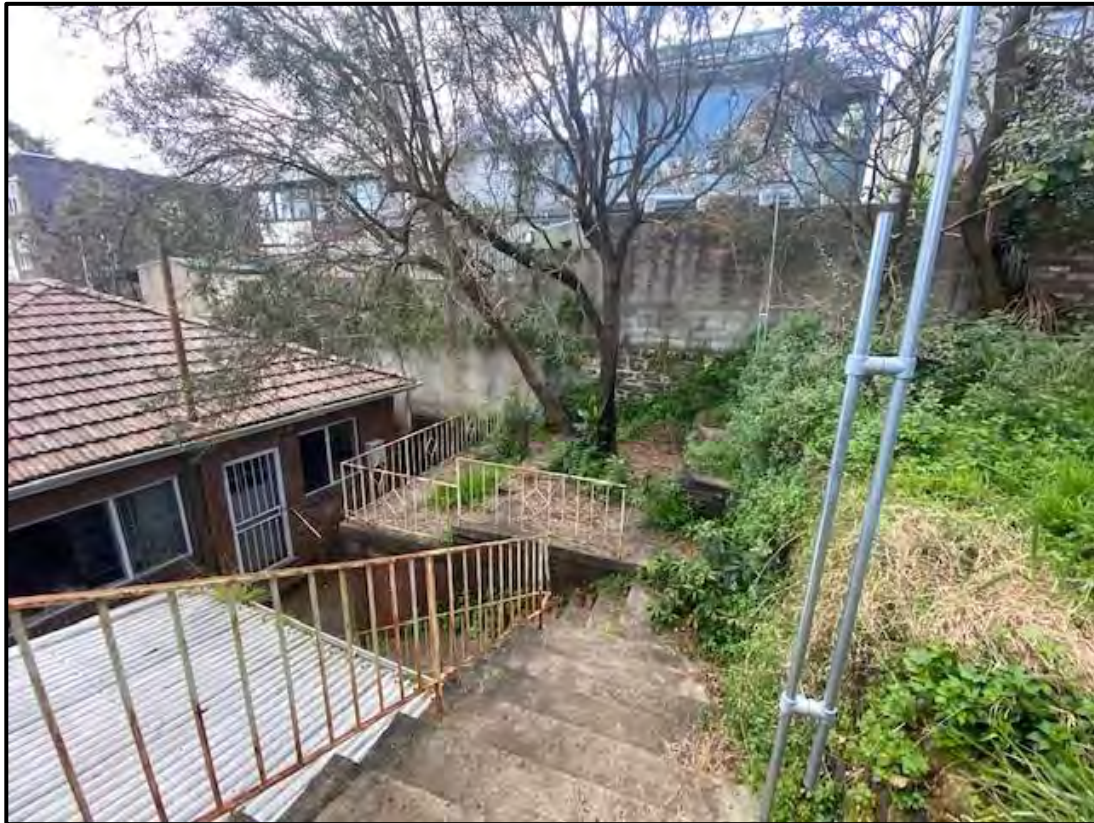
Figure 15: Rear of dwelling and existing built-up area and access stairs
