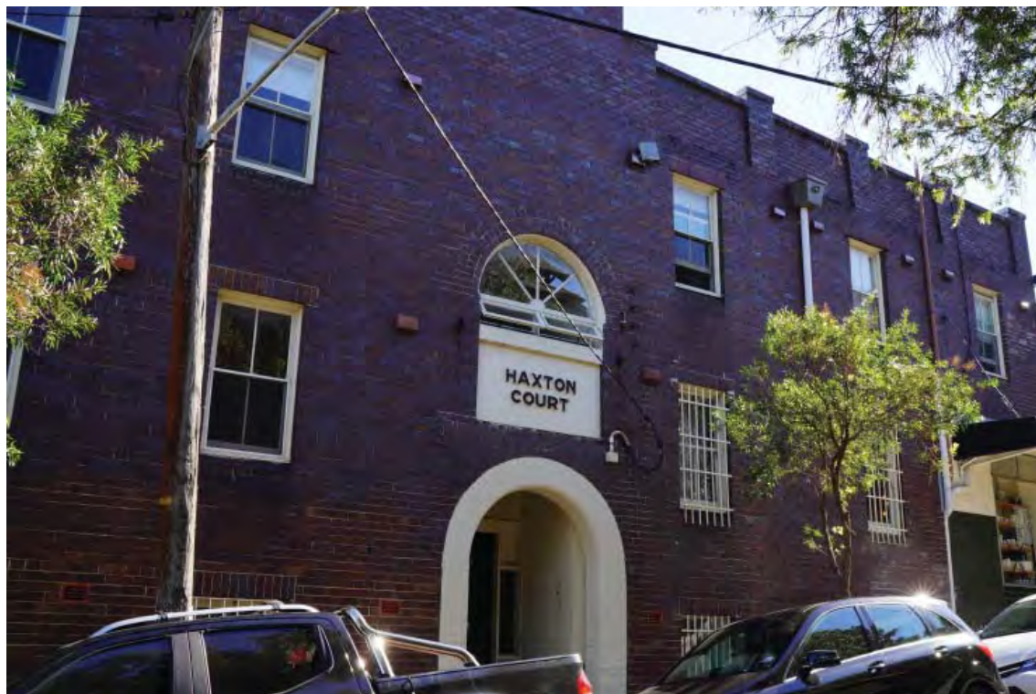
Plate 21 East elevation of Haxton Court viewed from Thomas Street
