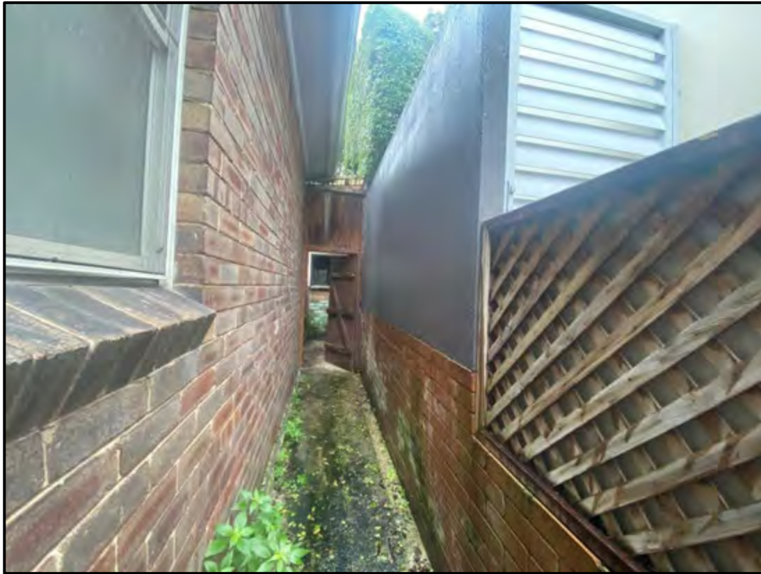
Figure 19: Existing paved path and fencing/walls along southern side setback – view towards rear yard
