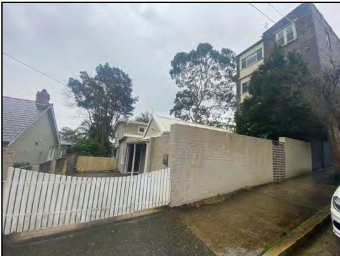
Figure 25: Front of dwelling house at No. 60 Thomas Street
