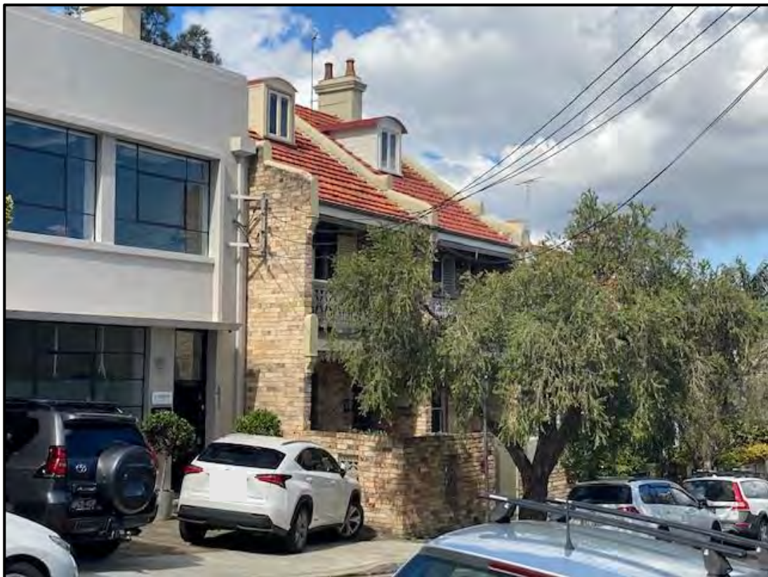
Figure 27: Front of semi-detached housing at No. 37 and 39 Thomas Street
