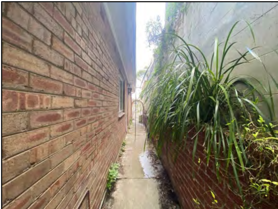
Figure 14: Existing paved path and fencing/walls along northern side setback
