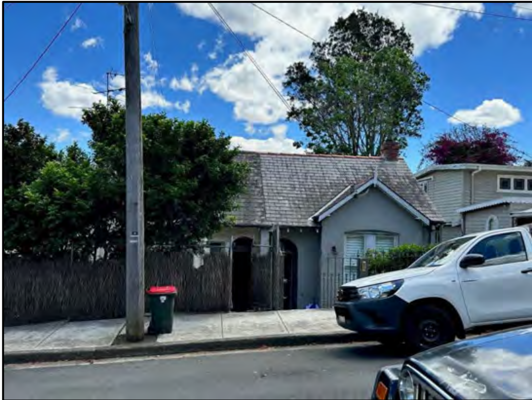
Figure 28: Front of semi-detached housing at No. 56 and 58 Thomas Street
