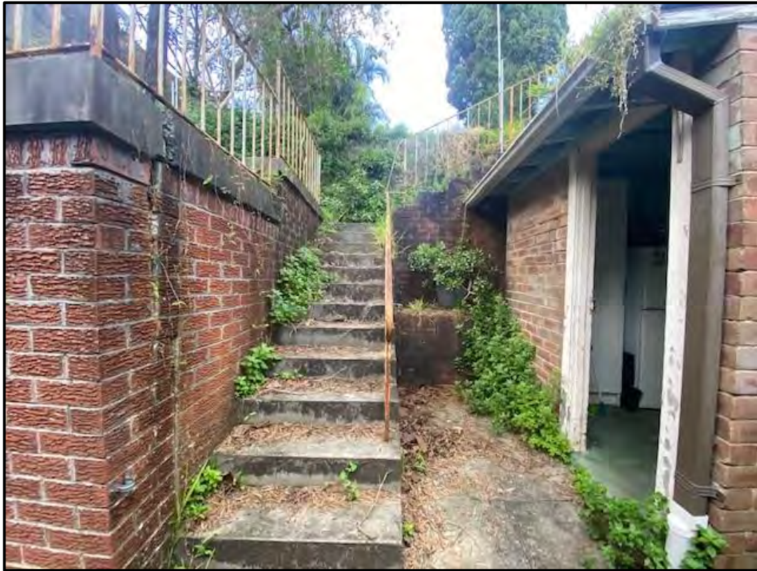
Figure 17: Access stairs leading to upper portions of rear yard
