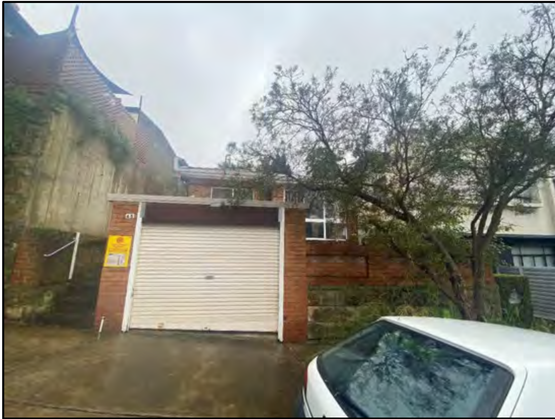
Figure 13: Closer view of the front setback of site
