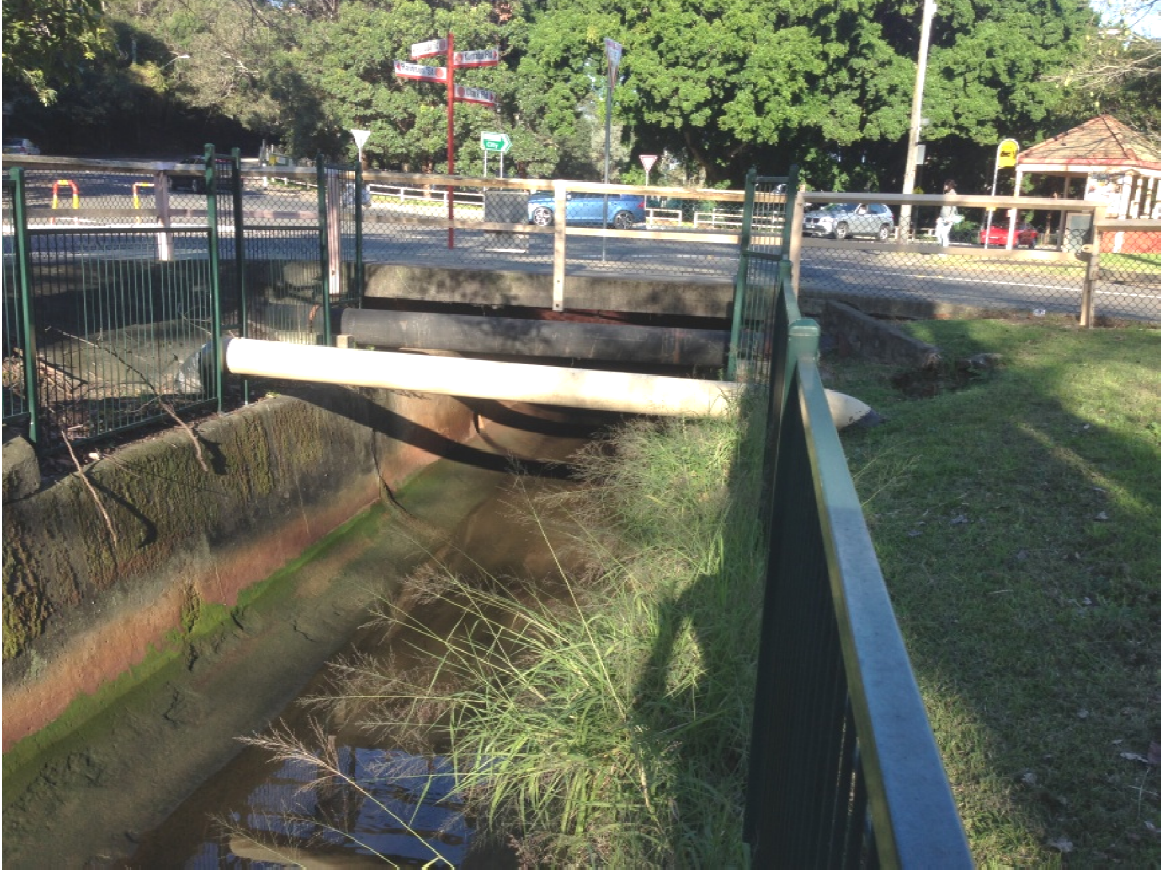
Above: Kurraba Road Culvert (18/06/2014)
