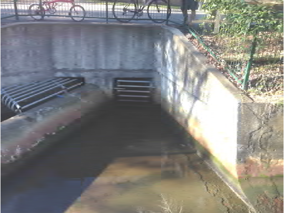
Above: CDS unit located at Junction of Rawson Street and Kurraba Road (18/06/2014)
