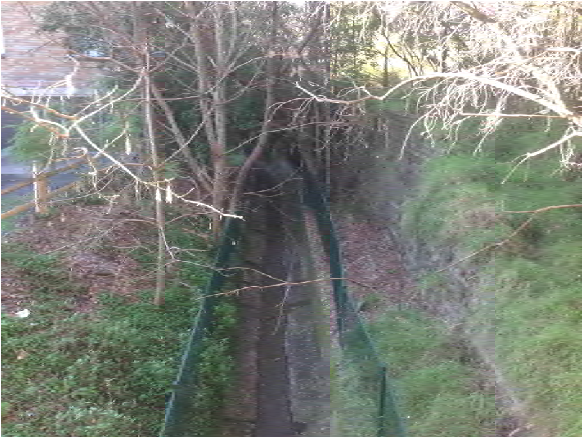
Above: Open Channel Downstream of Eaton Street (18/06/2014)
