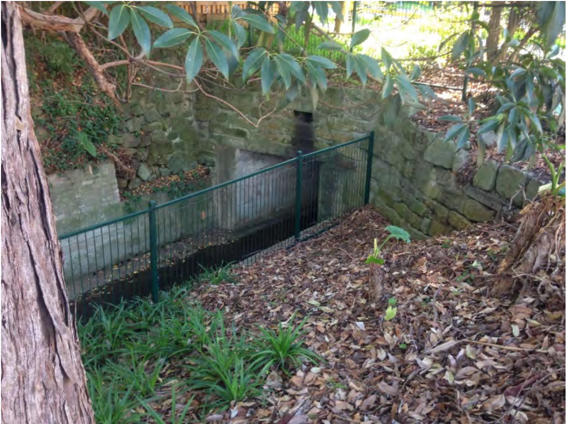
Above: Darley Street Culvert (18/06/2014)
