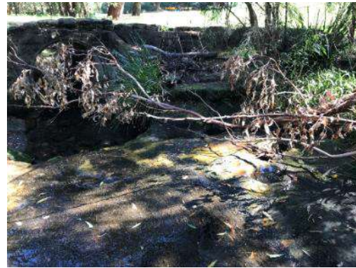
Storm issues, Northwood
