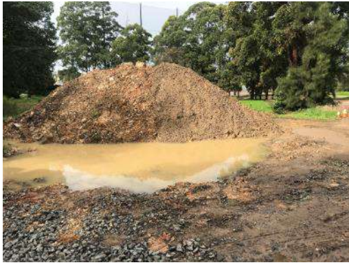
Works inspection, South Strathfield
