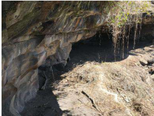
Excessive vegetation clearance, Cammeray
