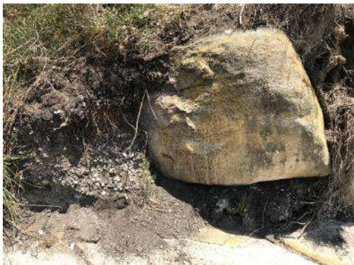
Coastal erosion monitoring, Northbridge
