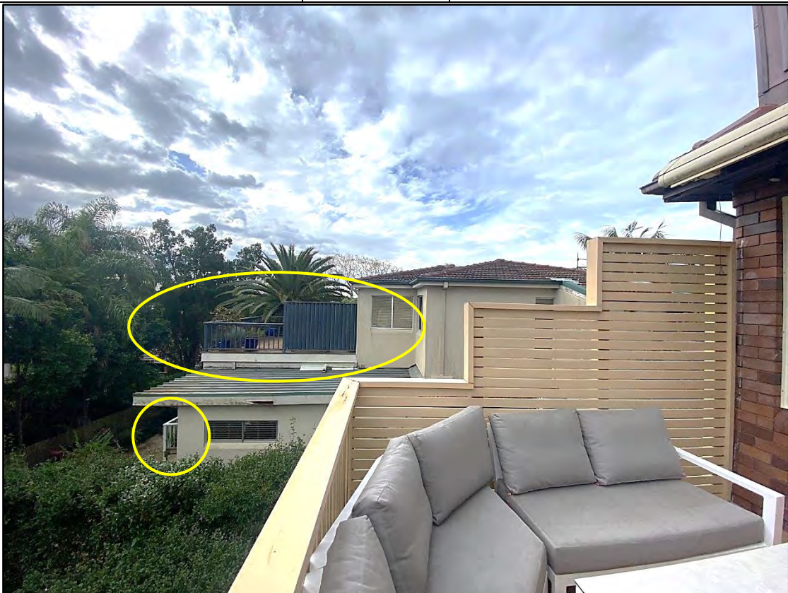
Figure 32: View of No. 46 Ellalong Road – existing elevated terrace/balcony areas (circled in yellow)
