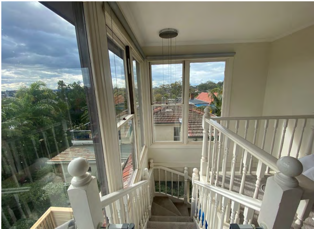
Figure 22: Existing stairwell taken from first floor of dwelling house
