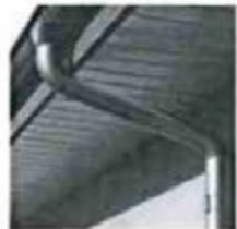
3 Half round metal gutter & downpipes
