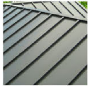
1 Metal Roofing Standing Seam
