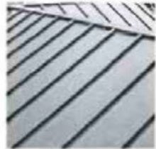
1 Metal Roofing Standing Seam
