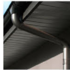
3 Half round metal gutter & downpipes
