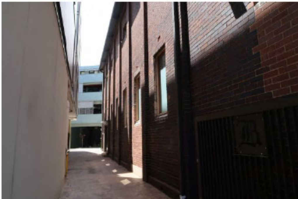
Figure 14: Northern passageway between the subject site and neighbouring development 319 Pacific Highway, view looking east (Source: NBR)
