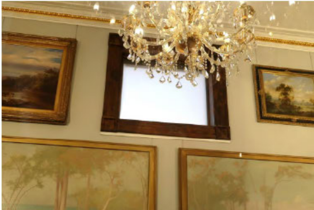
Figure 21: Elevated window within jeweller room in the ground floor foyer to be retained but infilled in the proposed works, view looking north (Source: NBR)
