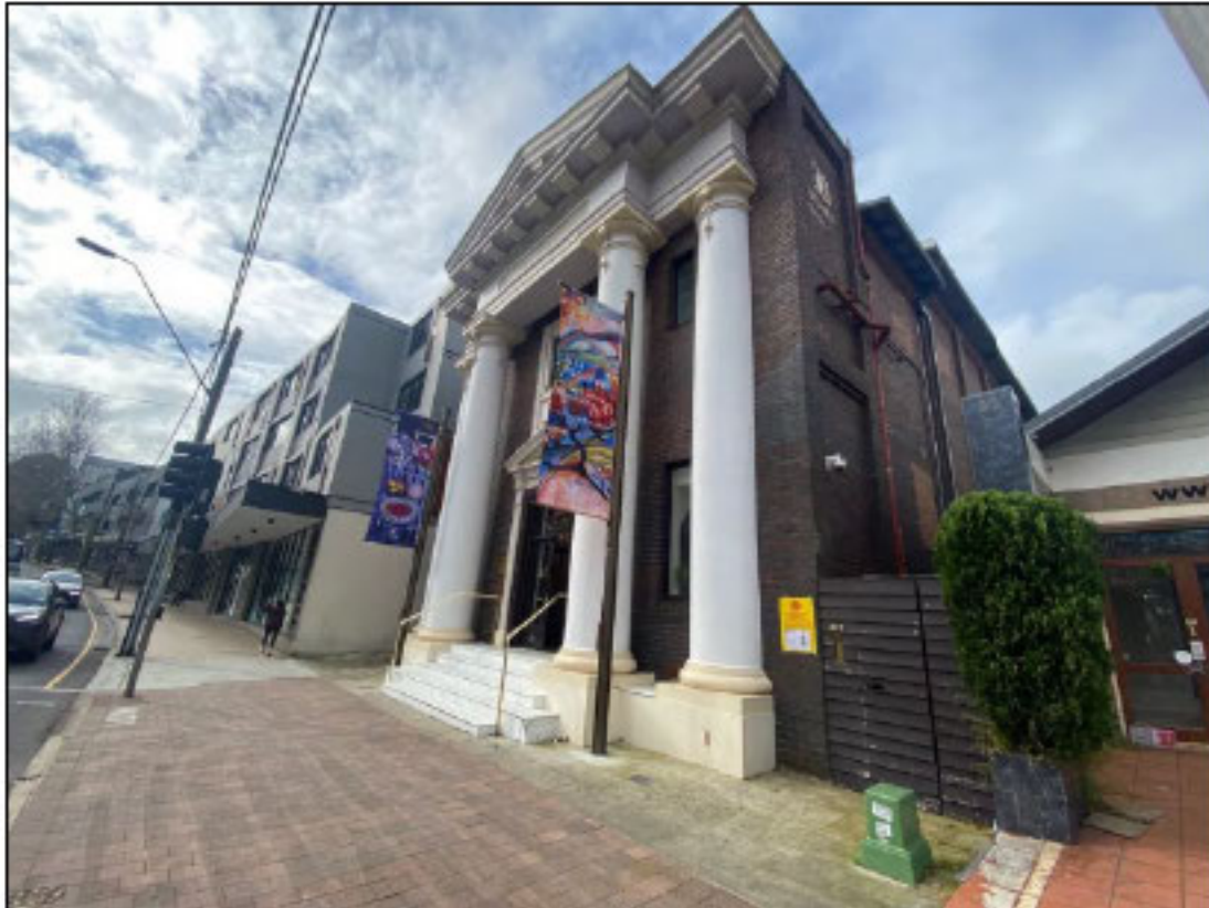
Figure 11: Front façade of existing building (Former Masonic Temple) within subject site.
