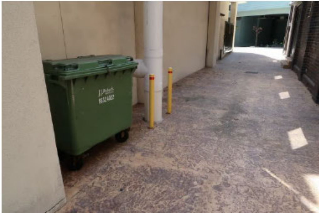
Figure 17: Slab covering the northern passageway beside the subject site, works will require installation of footings on the northside of the passageway to support the proposed first floor addition (Source: NBR)
