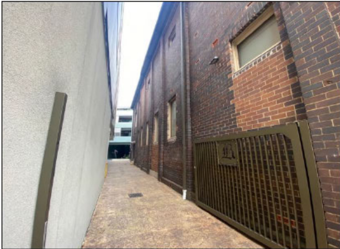
Figure 12: Northern side setback – paved passageway within subject site.
