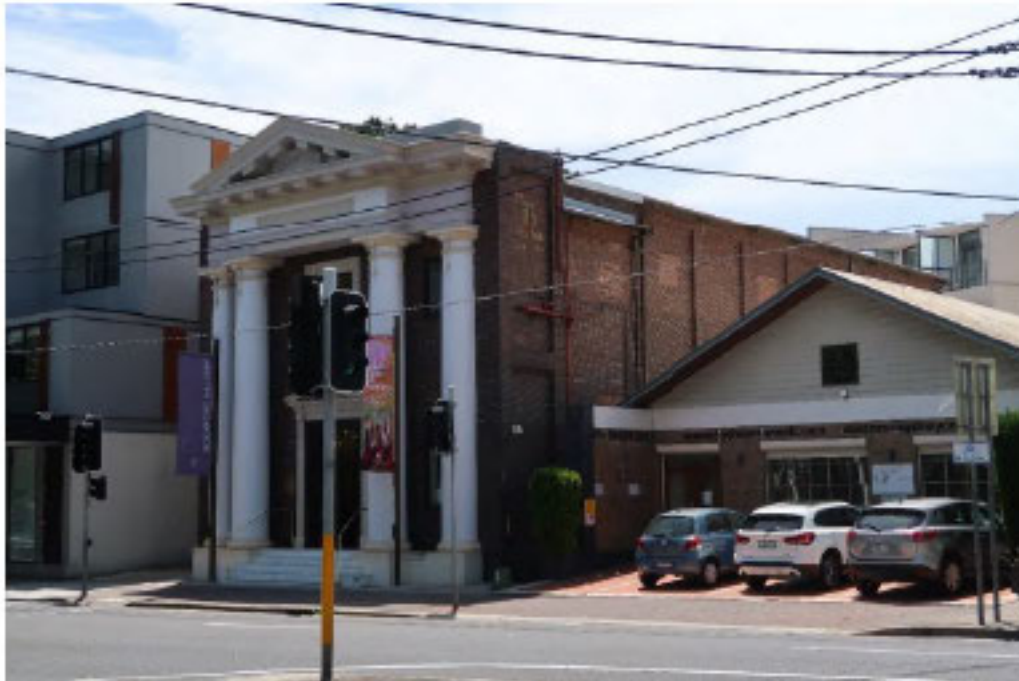
Figure 13: View to the exterior of the subject site looking northeast, blocked up windows on the first floor of the southern elevation visible (Source: NBR)
