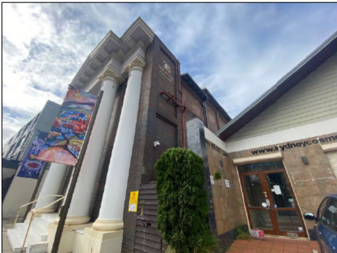
Figure 15: Southern side of existing building
