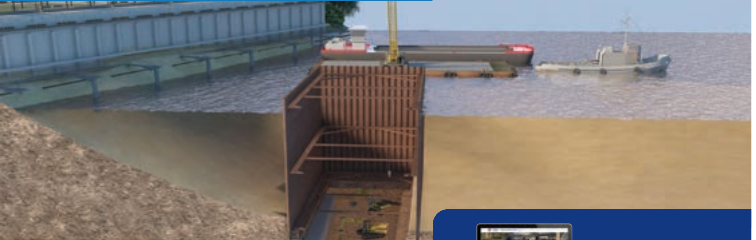
Artist's impression of cofferdam construction in Sydney Harbour
