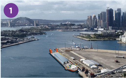
1 Construction and fitout of immersed tube tunnel units at White Bay
