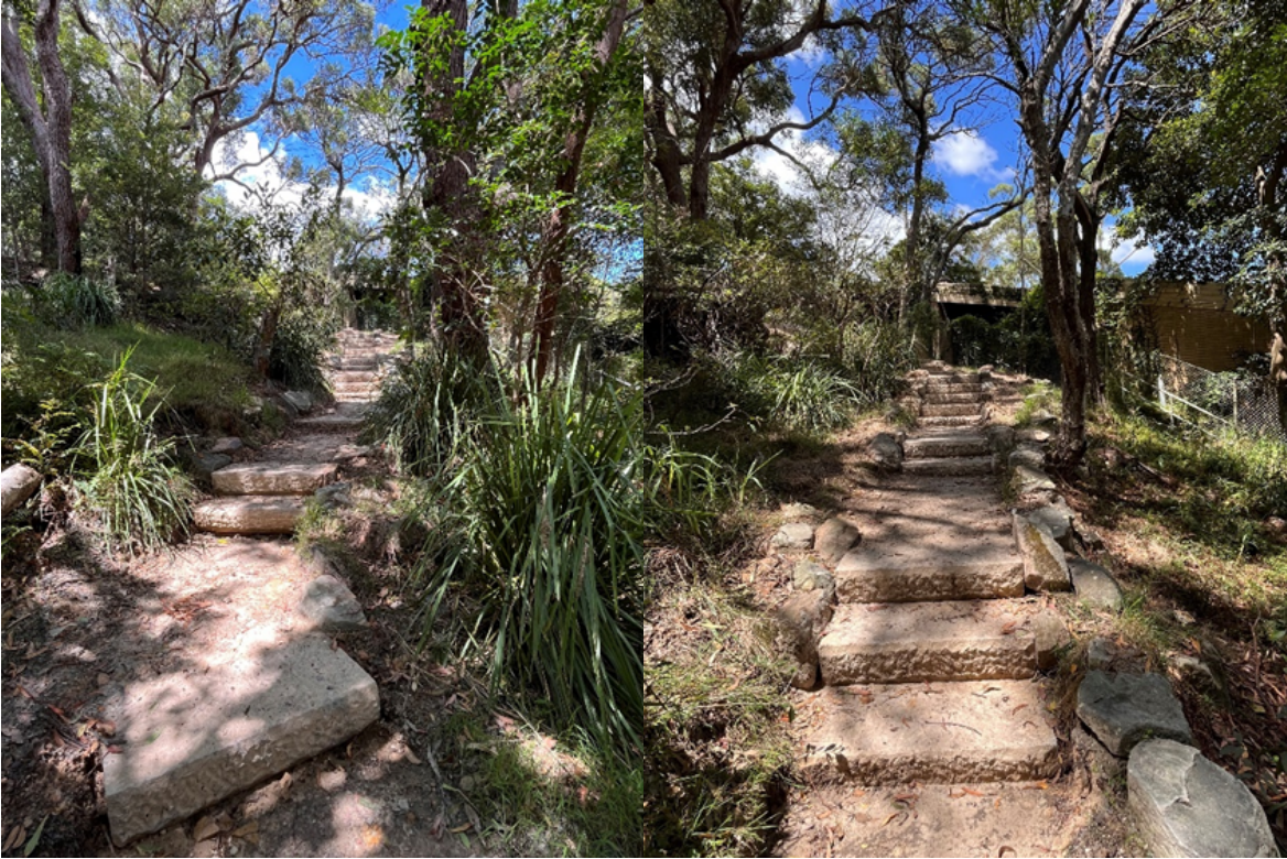
Above left & right: Hand-faced dimension sandstone steps replacing sleeper box steps
