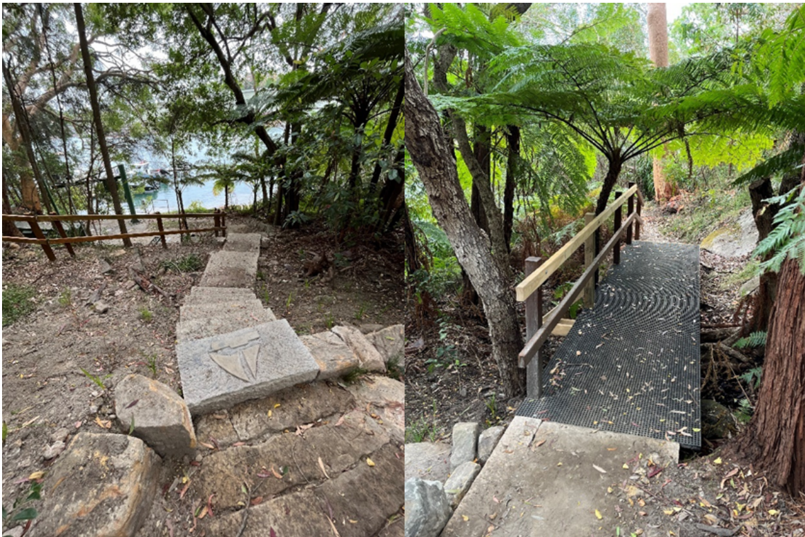
Above left: link track to foreshore with integrated drainage swale in foreground
