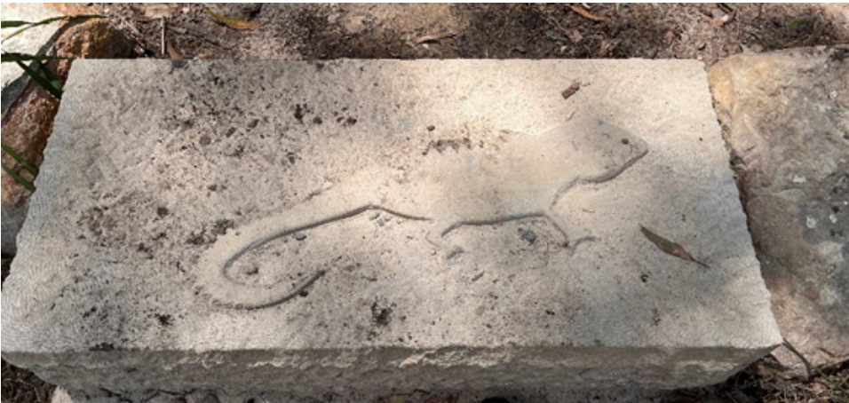
Above left & right: Hand-faced dimension sandstone steps replacing sleeper box steps
