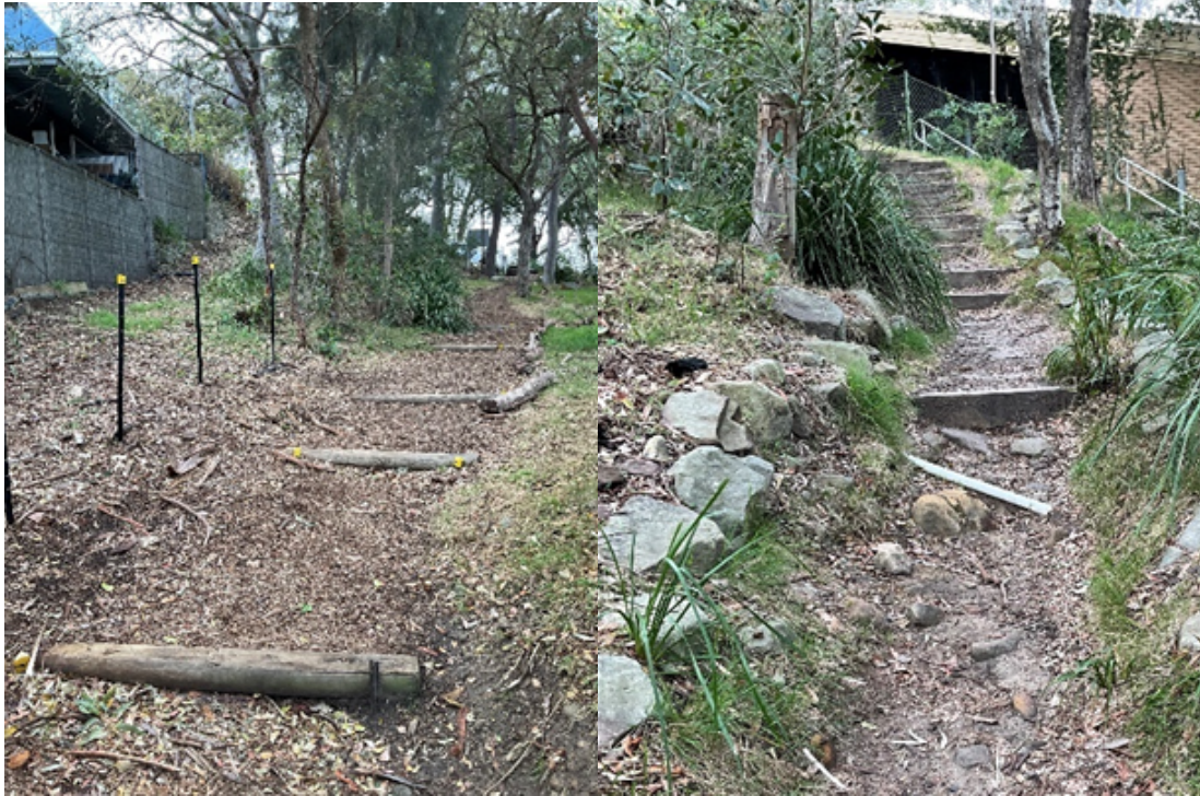
Above left: Treated pine log steps with exposed steel pickets
