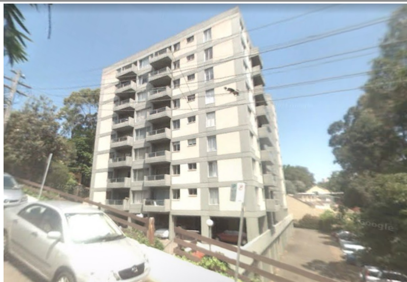
Figure 2: View of site from French Street Source (Google StreetView)
