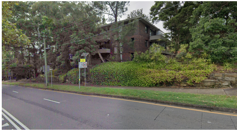
Figure 4: View of site from Miller Street Source (Google StreetView)
