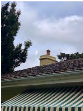
Figure 3. 64: Chimney and roof pan tiles
