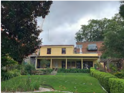
Figure 3. 110: Former garage and flatette
