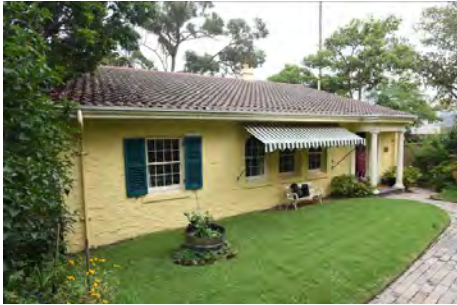
Figure 3. 59: Front (eastern) elevation
