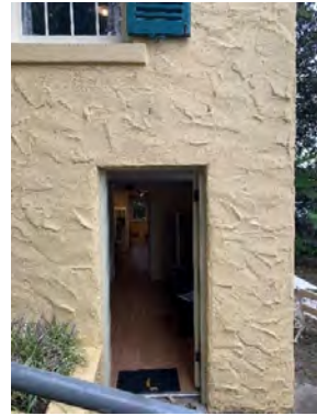
Figure 3. 73: Entry into former Laundry in the lower level
