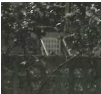
Figure 7. 2: Detail from a 1930s photograph of Nutcote looking westward towards Wallaringa Road. The original or early timber slat gate is visible. Source: Stanton Library
