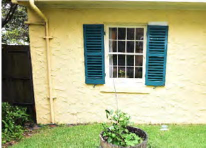
Figure 3. 62: Typical multipaned sash window with shutters
