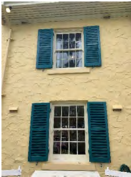
Figure 3. 68: Windows on west elevation with shutters
