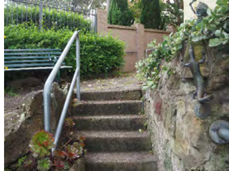
Figure 3.36: 3.37: Concrete and stone steps with metal handrails connecting House Terrace to Lower Garden with rockeries.
