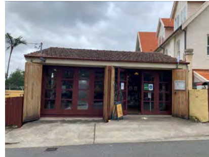
Figure 3. 111: Street elevation of the Garage
