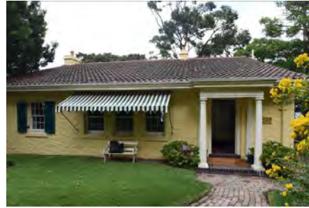
Figure 3. 60: Front (eastern) elevation, showing entry portico.
