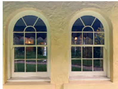
Figure 3. 63: Detail of multipaned round headed sash windows.
