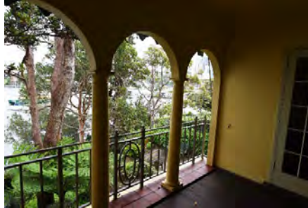
Figure 3.95: Loggia with door from Dining Room
