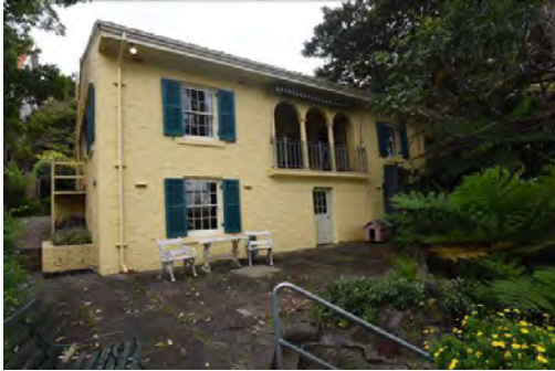
Figure 3. 66: Rear (western) elevation
