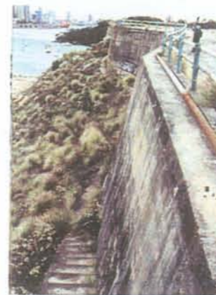
Dramatic battered concrete walls
