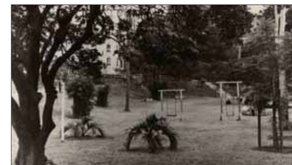
Figure 17 Watt Park, North Sydney c.1937 (source: Stanton Library)
