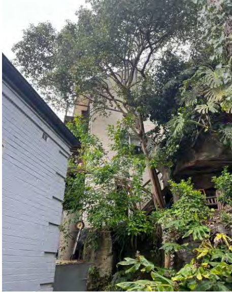
No. 3 East Ave – part 3 storeys
