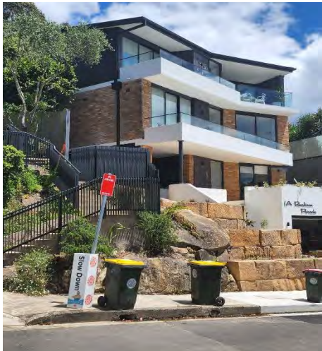
No. 7 Rowlinson Pde– 3 storeys
