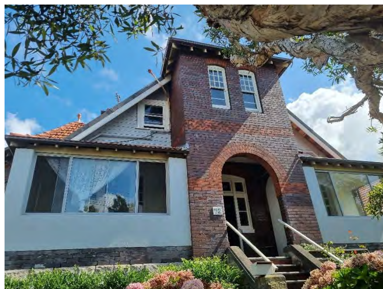
Figure 8. Site Photo of Kurraba Road elevation
