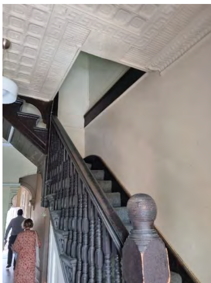
Figure 11. Site photo of existing internal staircase and features
