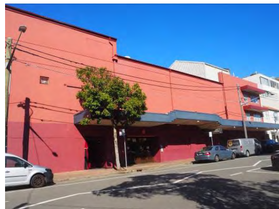
Figure 3. 66: Rear of the Cinema, viewed from Parraween Street.
