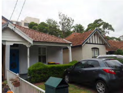
Figure 2. 93: Frontage of No. 80 Parraween Street with No. 82 Parraween Street adjacent.
