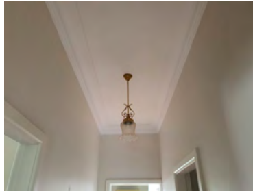
Figure 2. 118: Cornices to hallway.
