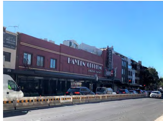
Figure 3. 54: Straight-on view of the Cinema from Military Road
