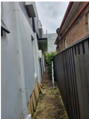
Figure 2. 46: Side passage showing east elevation.
