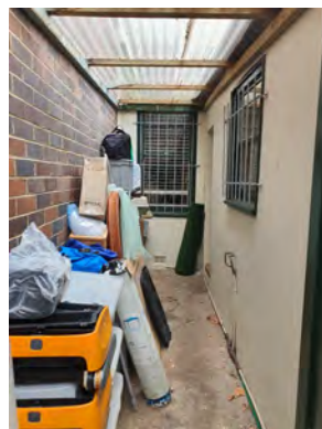
Figure 2. 31: Side passage with window to main wing.
