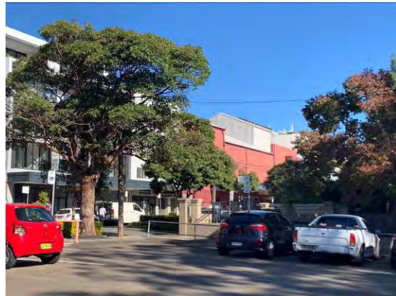
Figure 3. 60: View towards the rear elevation of the Cinema from Parraween Street carpark.
