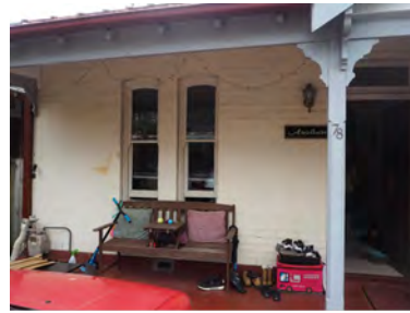
Figure 2. 77: Front elevation of No. 78 Parraween Street.
