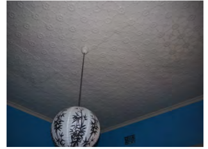
Figure 2. 86: Pressed metal ceiling in second bedroom.
