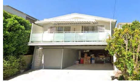
Figure 3. 17: The rear development to No. 78 Gerard Street. Source: Google Streetview
