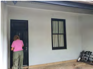
Figure 2. 43: Front elevation with later addition window, front door and sandstone paving to verandah.
