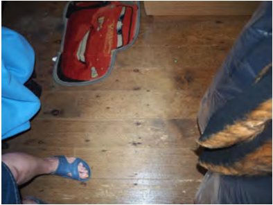
Figure 2. 84: Original timber flooring in front bedroom.
