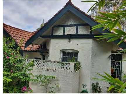
Figure 3. 43: Front elevation of No. 14 Macpherson Street.
