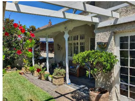
Figure 3. 65: North elevation of No. 42 Boyle Street.
