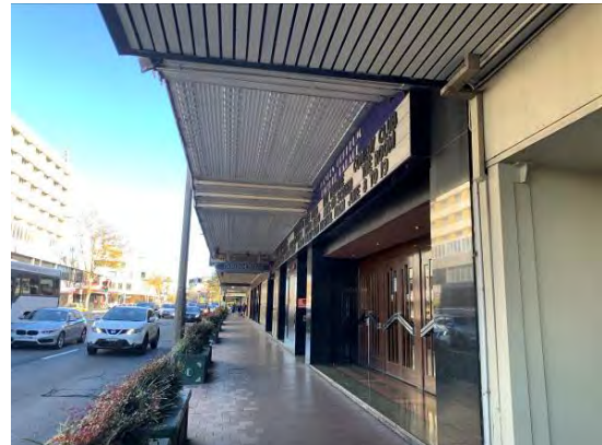
Figure 3. 64: Awning over original entry foyer, looking west.
