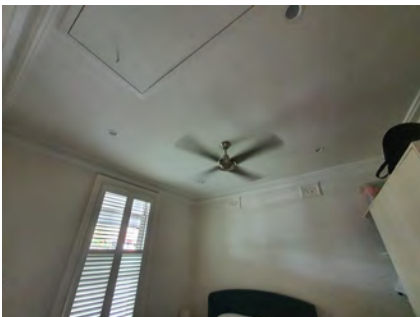
Figure 2. 25: Ceiling to bedroom with original cornices.
