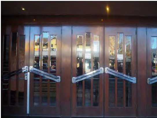
Figure 3. 63: Entry doors to original foyer (possibly original).
