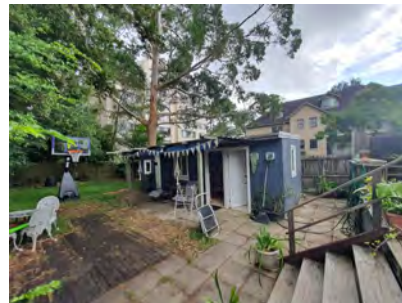
Figure 2. 145: Shed located in rear yard.
