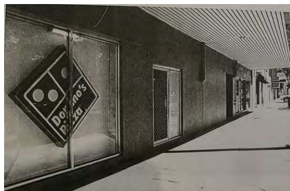
Figure 2. 52: Rear façade (Parraween Street) in 1998. Source: Rod Howard Heritage Conservation, March 1998
