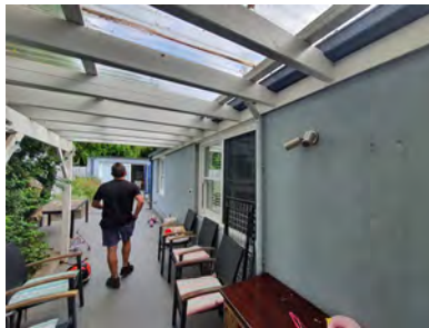
Figure 2. 17: Side passage with portico.
