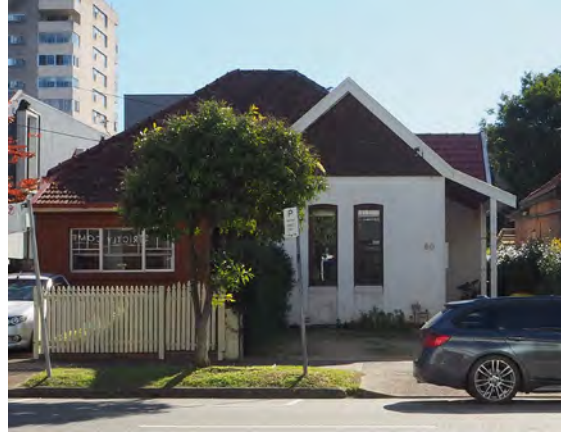
Figure 3. 19: Nos. 58 & 60 Parraween Street.
