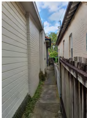
Figure 2. 112: View down west side passage.
