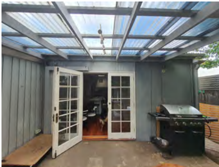
Figure 2. 51: Rear elevation of rear wing.
