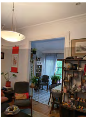
Figure 2. 154: Altered door opening to dining room.
