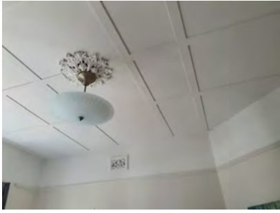
Figure 2. 130: Battered ceiling with ceiling rose and picture rail to master bedroom.
