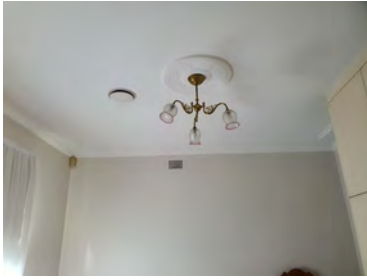
Figure 2. 117: Ceiling and cornices to master bedroom.
