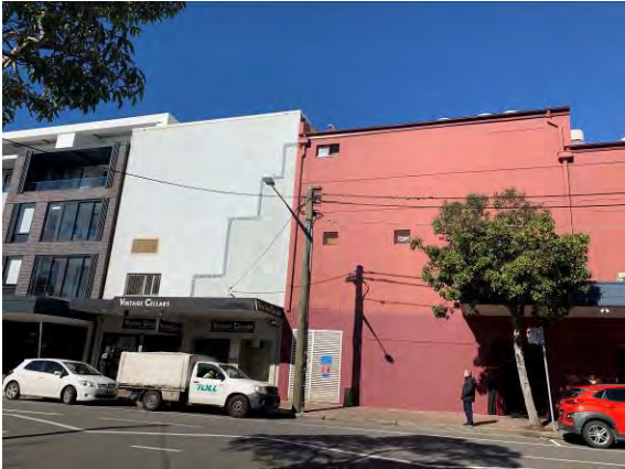
Figure 3. 67: Eastern side of the rear of the Cinema. The adjoining building painted white now forms part of the complex.
