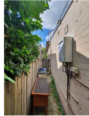
Figure 2. 94: Side passage to east side of house.
