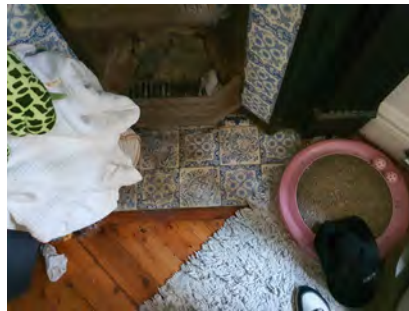
Figure 2. 134: Detail of tiling to living room fireplace.
