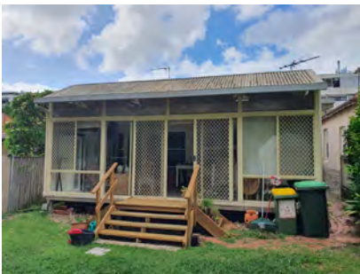
Figure 2. 111: Rear elevation of rear wing.
