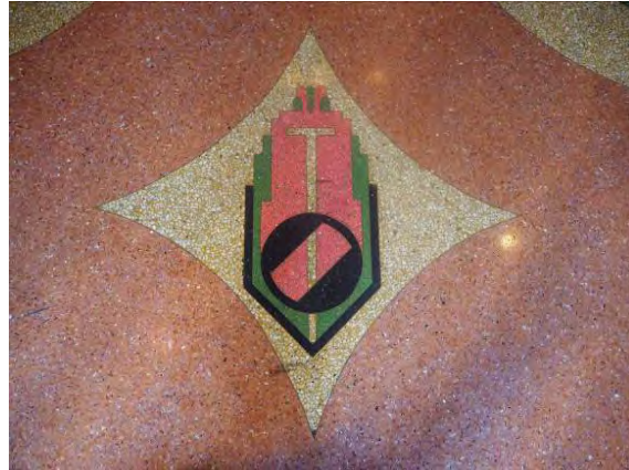
Figure 3. 74: Original decorative terrazzo motif on floor of original foyer.
