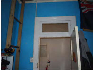
Figure 2. 85: Typical internal door with fanlight to second bedroom.
