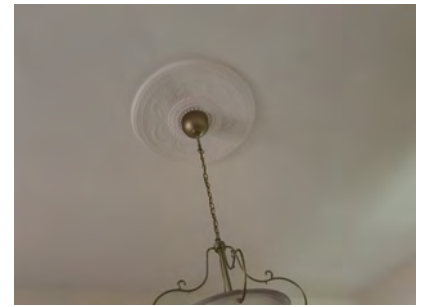
Figure 2. 135: Ceiling rose to living room.
