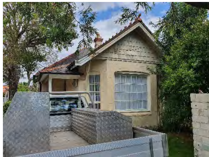
Figure 3. 24: No. 28 Macpherson Street.
