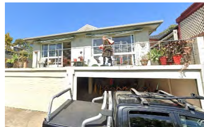
Figure 3. 13: The rear development to No. 74 Gerard Street. Source: Google Streetview
