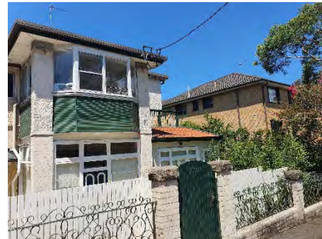
Figure 3. 57: The southern half of No. 21 Murdoch Street.
