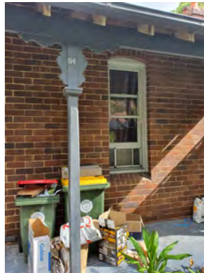
Figure 2. 126: Verandah post and bracket, exposed eaves rafters and front window.
