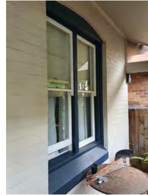
Figure 2. 110: Original windows to front elevation.
