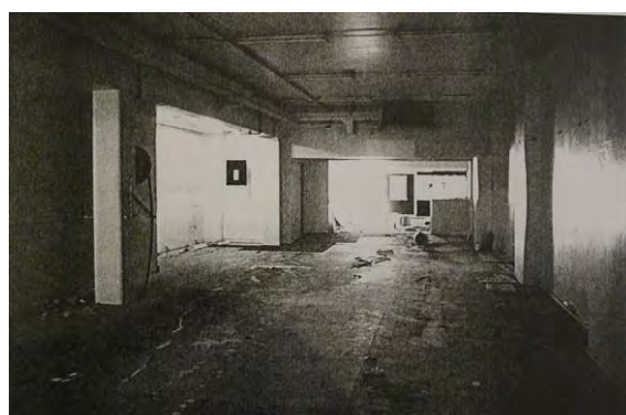
Figure 2. 54: Western-most shop to the ground floor. Source: Rod Howard Heritage Conservation, March 1998
