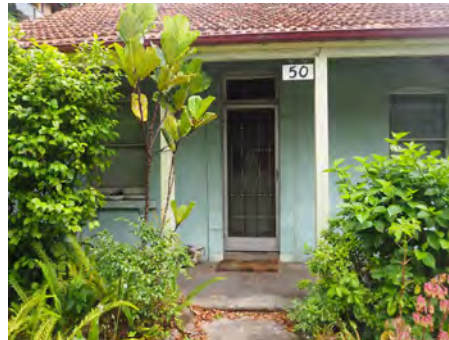
Figure 2. 2: No. 50 Parraween Street front door detail.
