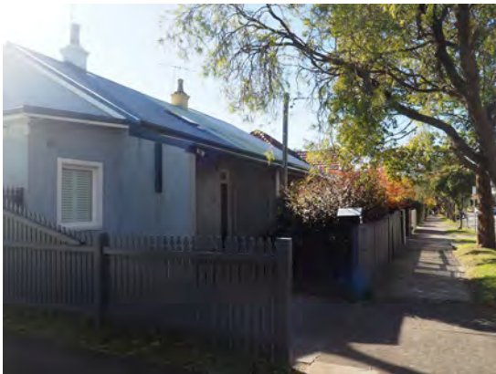
Figure 3. 17: Nos. 52 to 56 Parraween Street, a row of attached workers cottages dating from c.1889.
