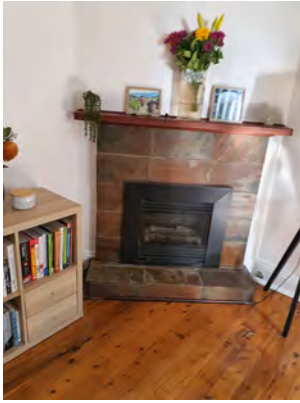
Figure 2. 103: Later addition fireplace and hearth to original chimney breast in living room.
