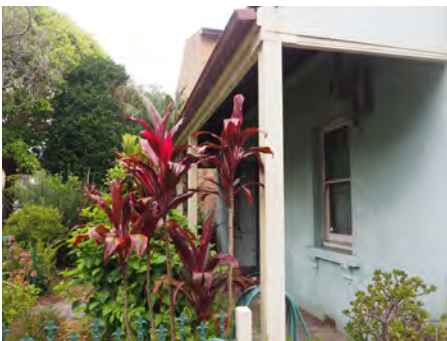
Figure 2. 3: Detail of front verandah and window
