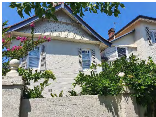
Figure 3.54: Northern half of No. 23 Murdoch Street.
