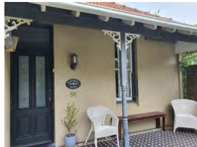
Figure 2. 143: Front verandah and front door.
