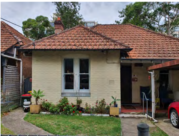
Figure 2. 141: Front elevation of No. 86 Parraween Street.
