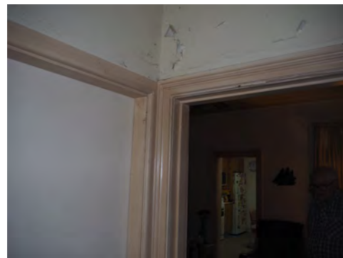
Figure 2. 10: Typical internal architraves.
