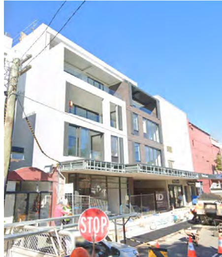
Figure 3.96: The rear elevations of No. 390-394 Military Road, as seen from Parraween Street.
