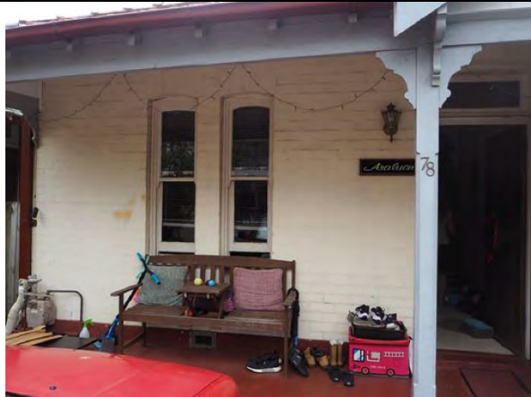
FIGURE 20: Front elevation of No. 78 Parraween Street, Cremorne
