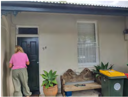
Figure 2. 27: Front elevation of No. 54 Parraween Street
