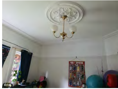
Figure 2. 147: Ceiling to master bedroom with ceiling rose, cornices and picture rail.
