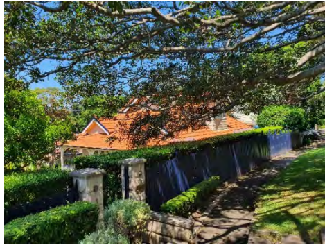
Figure 3. 75: No. 3 Iredale Avenue.
