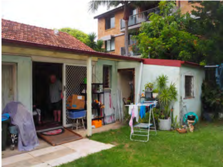
Figure 2. 7: Rear elevation with skillion addition.
