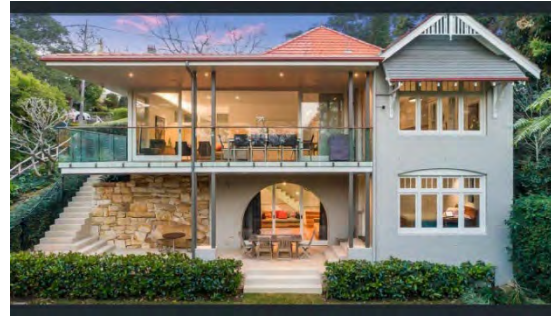
Figure 3. 78: Rear of No. 5 Iredale Avenue. Source: realestate.com
