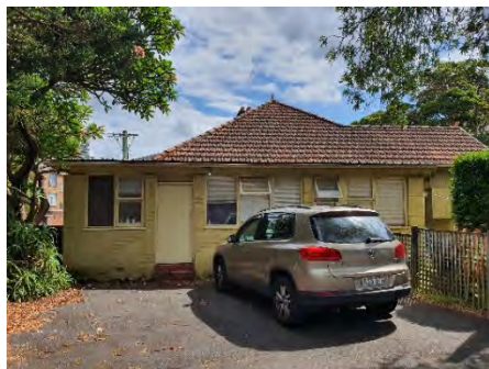
Figure 3. 35: South (side) elevation of No. 4 Macpherson Street.
