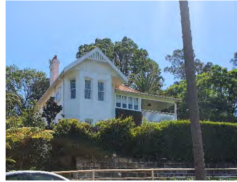
Figure 3. 70: No. 28 Iredale Avenue as seen from street level.
