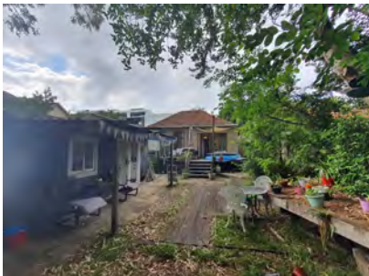
Figure 2. 144: View of rear yard and rear elevation.
