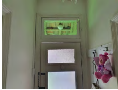
Figure 2. 140: Coloured glazing to front door fanlight.
