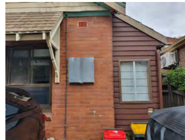
Figure 2. 62: Enclosed side verandah and original timber awning with brackets to front window (replaced with aluminium framed window).
