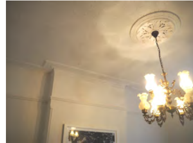
Figure 2. 72: Detail of original cornice, picture rail and ceiling rose to living room.
