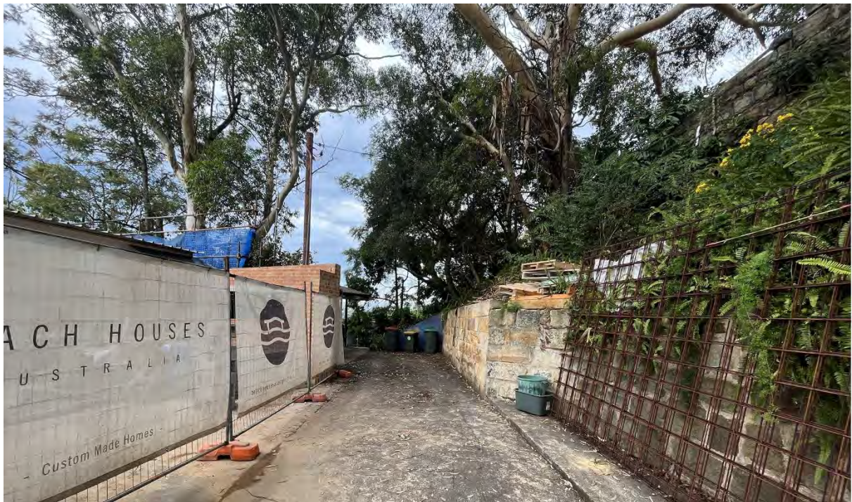
Figure 33: View of Cowdroy Avenue road reserve fronting No.56 and No.58 Cowdroy Avenue
