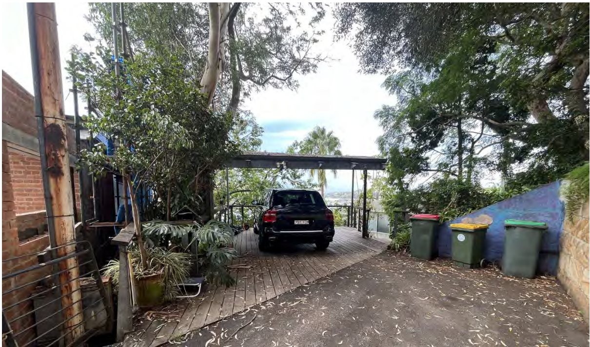
Figure 20: Photo of the site as viewed from Cowdroy Avenue. Asphalt surface is the public road pavement of Cowdroy Ave. Bins are placed in the Council road reserve. Existing retaining wall is proposed to be demolished and the road extended further along the street boundary.
