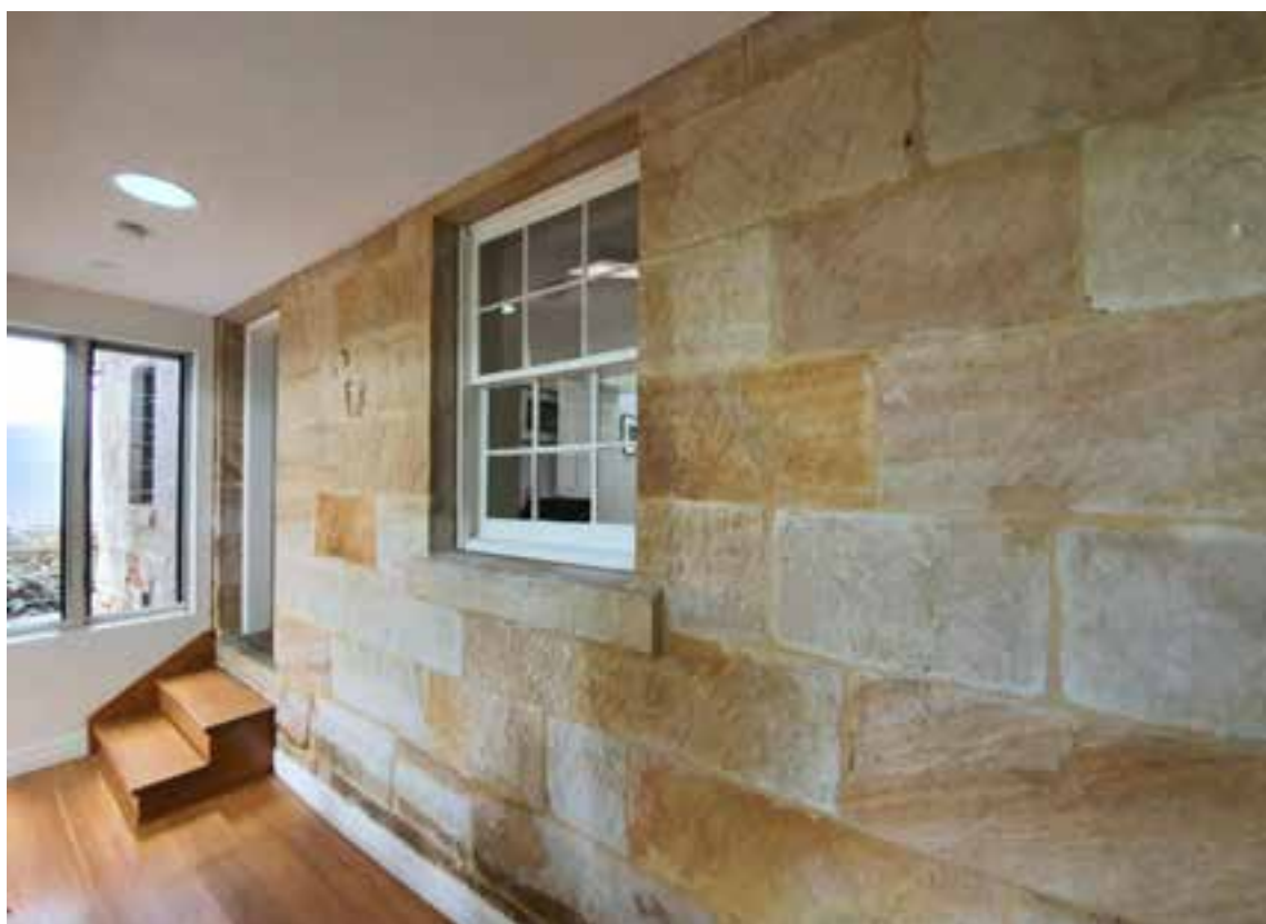
Figure 16: Rear sandstone wall of cottage
