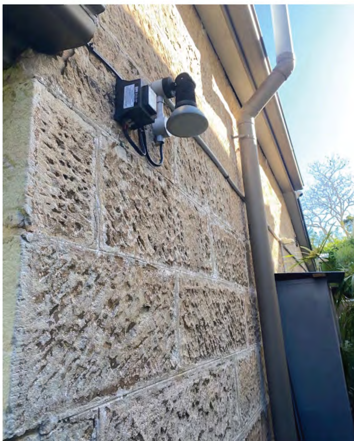
Eastern elevation of the sandstone cottage, facing north. Concave joint.
