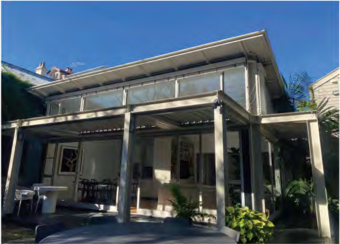
View to the rear wing from the backyard.
