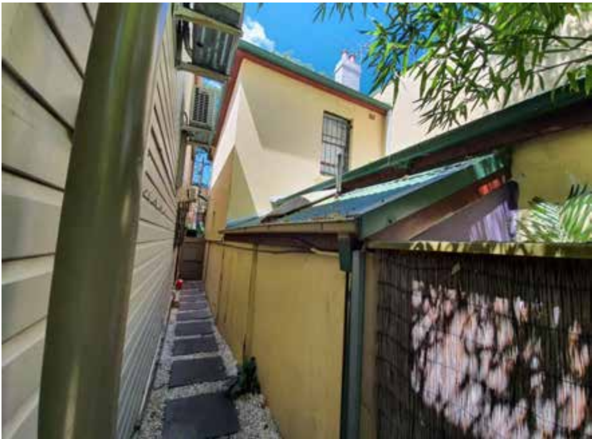
Figure 30: Existing western side path
