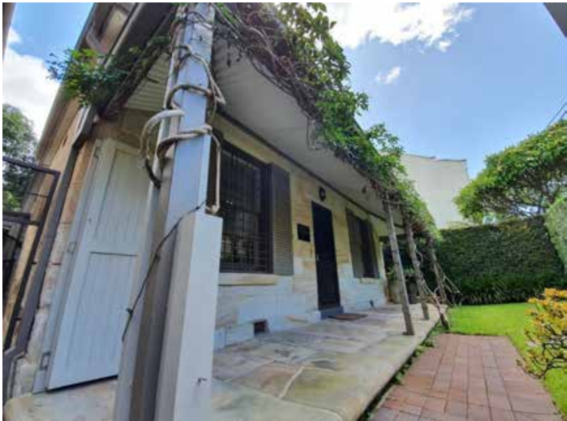
Figure 15: Existing sandstone cottage on Lot 3
