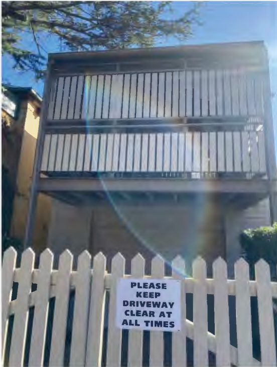
View to the side (west) garage/studio from the front path.
