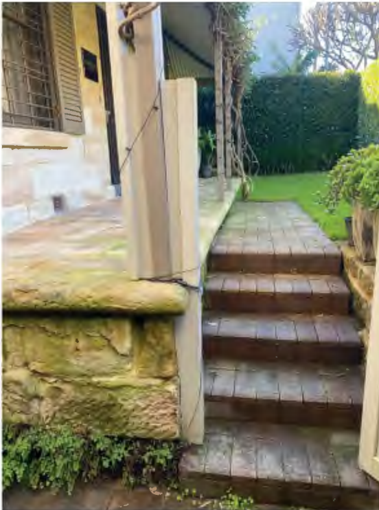
Non-original brick stairs and paving in front of the cottage's verandah.
