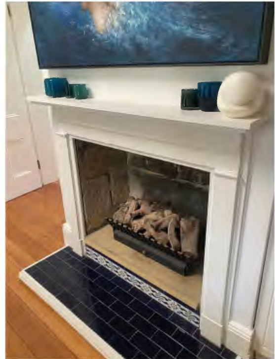
Study, fireplace with non-original tiled threshold. Timber mantelpiece and imposed pilaster surrounds are non-original.
