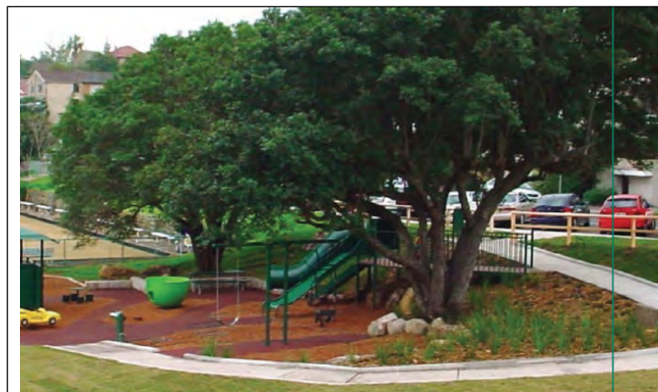
Concrete access ramp: Merrett Playground, Waverton
