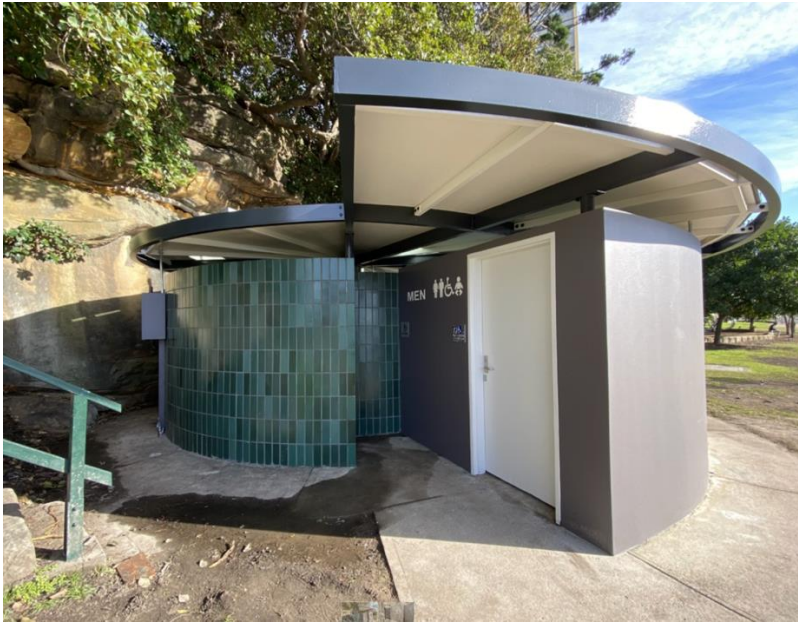
Amenities block – Blues Point Reserve, McMahon's Point
