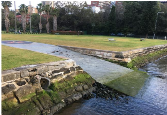
Milson Park boat ramp is now longer, wider and the slope is less steep
