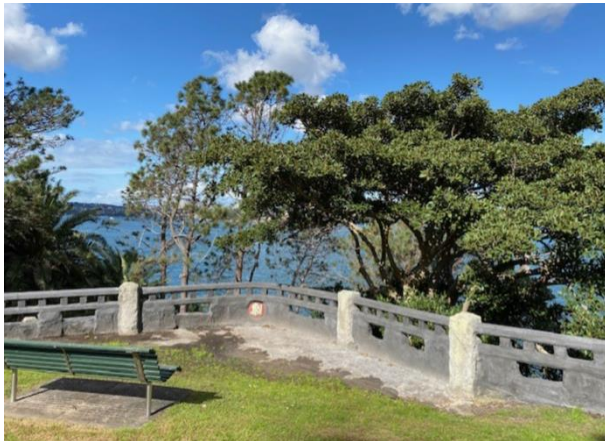
Repair of heritage depression-era fencing, and associated landscape works
