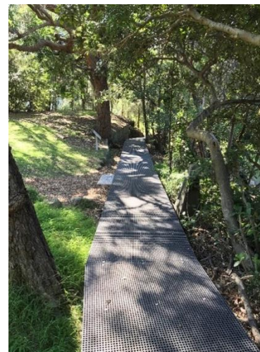
A new floating boardwalk protects an eroding shell midden
