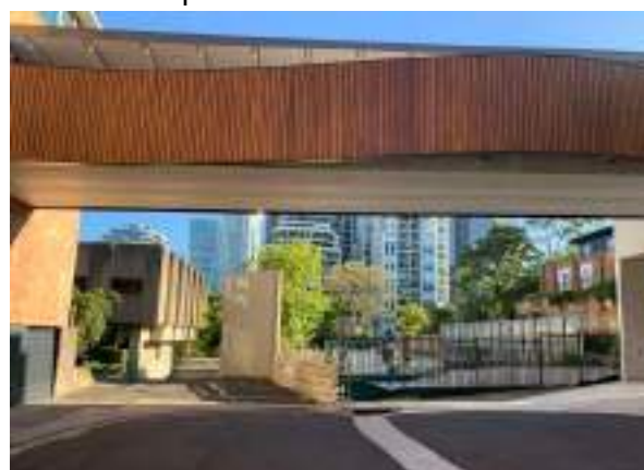
Figure 12 Overpass bridge connecting Wenona school campus
