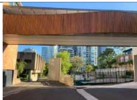
Figure 15: Overpass bridge connecting Wenona school campus
