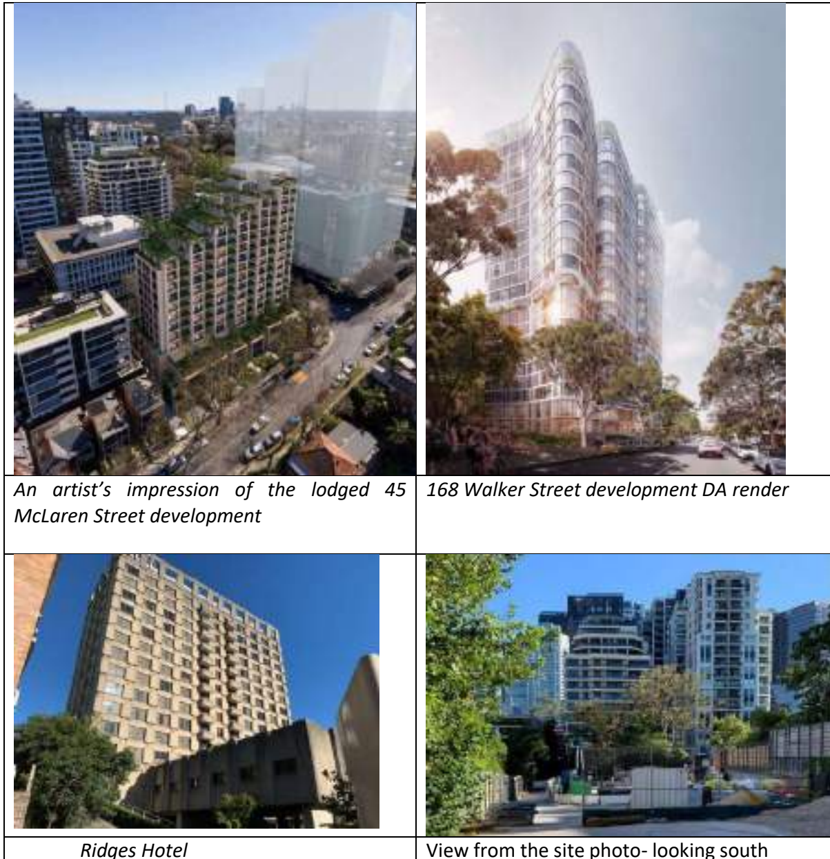
Figure 10: Evolving character and future built forms within the vicinity of the site
