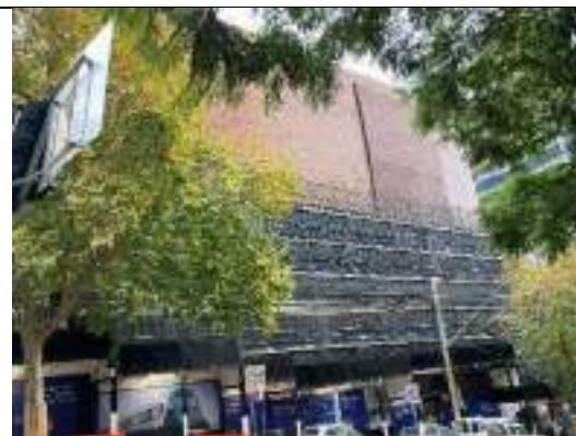
Figure 21: Victoria Cross North Portal
