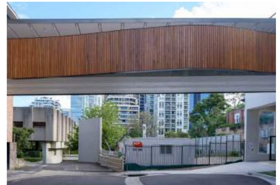
4. View south from Elliot Street with Wenona School footbridge in foreground
