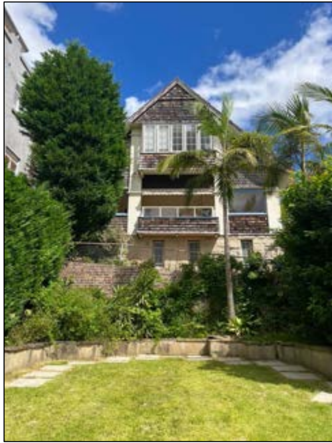
Photo 3: View of existing eastern elevation
