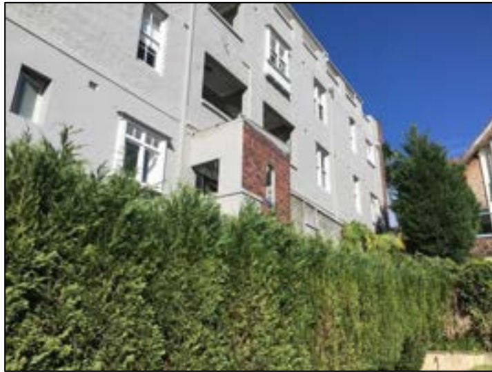
Photo 11: Northern elevation of No 11 Shellcove Road as viewed from subject site
