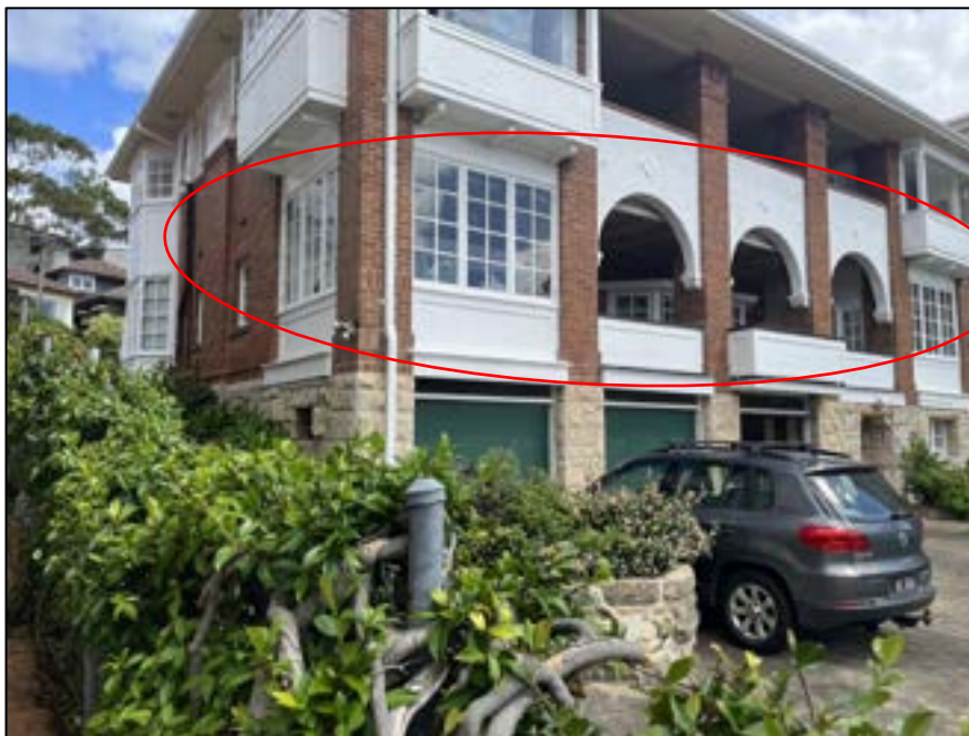
Photo 18: Location of Unit 1 of No 15 Shellcove Road outlined in red
