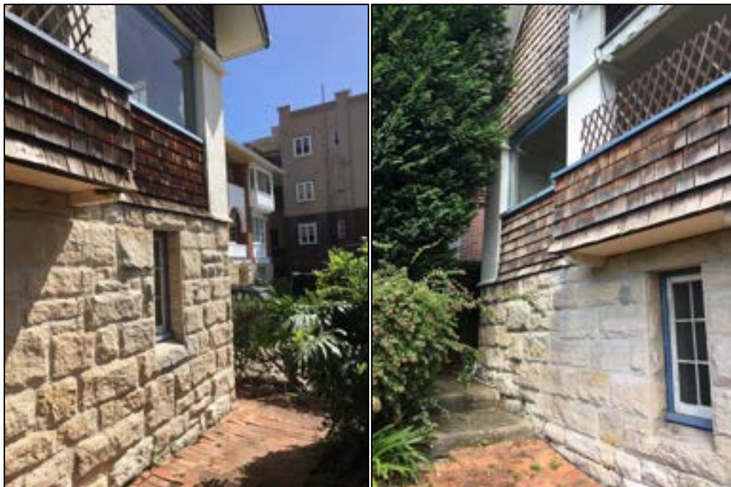
Photo 4: Existing Sandstone base at rear of dwelling
