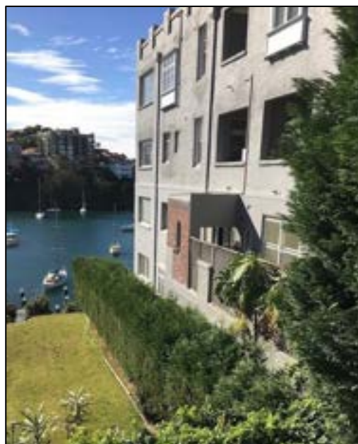
Photo 19: Northern elevation of No. 11 Shellcove Road
