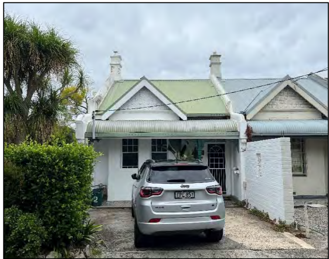
Figure 8. Southern elevation of the subject site viewed from Byrnes Avenue.
