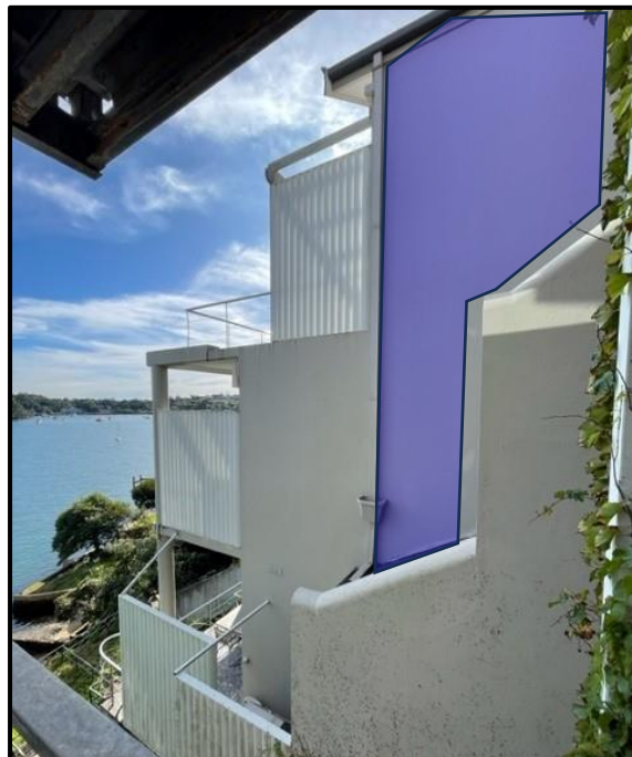
Figure 2: Existing southern elevation of subject dwelling with portion of new southern wall (shaded in blue) that will be close to the boundary and behind the current parapet wall
