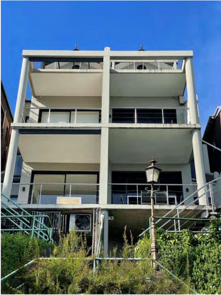
View of rear of existing
