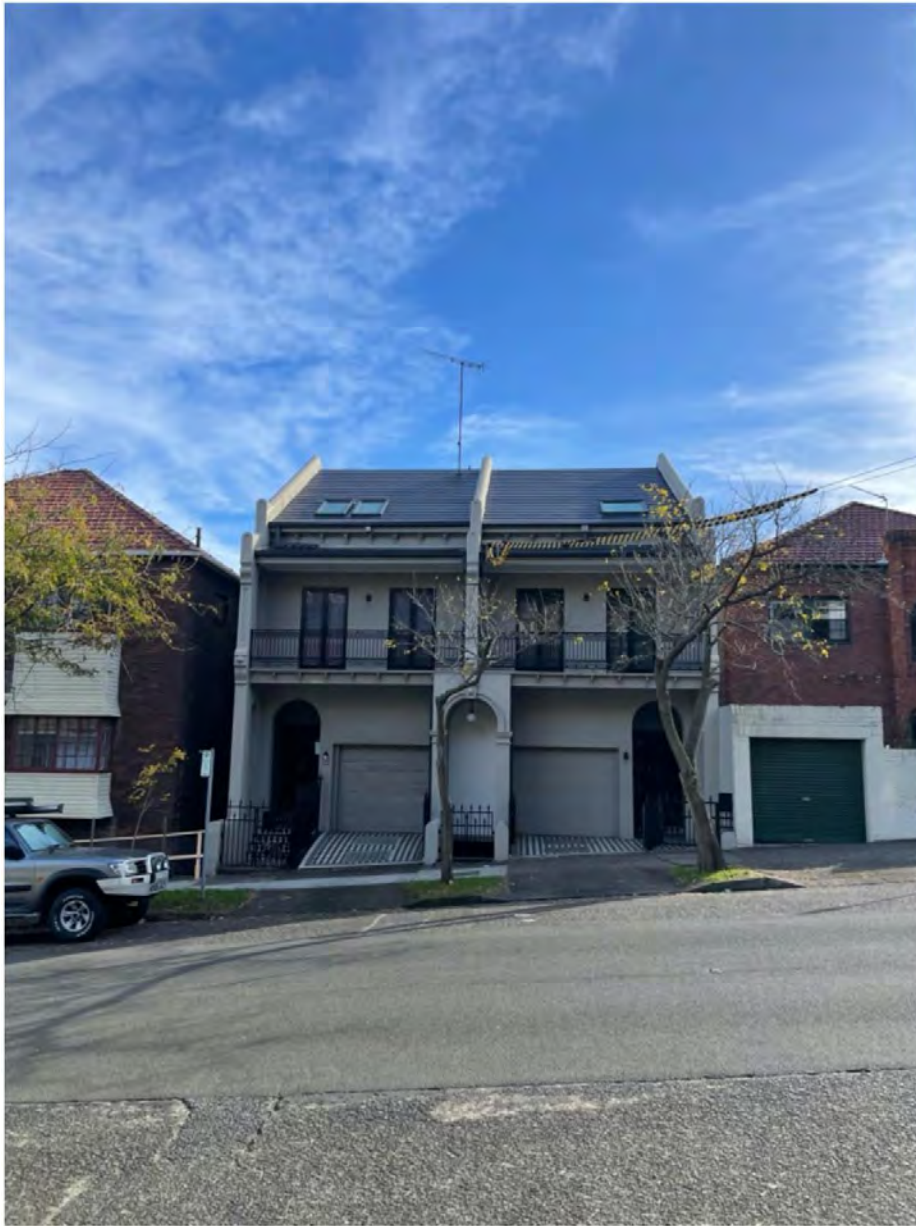
Neighbouring Inter-war flat buildings either side of existing (on left)
