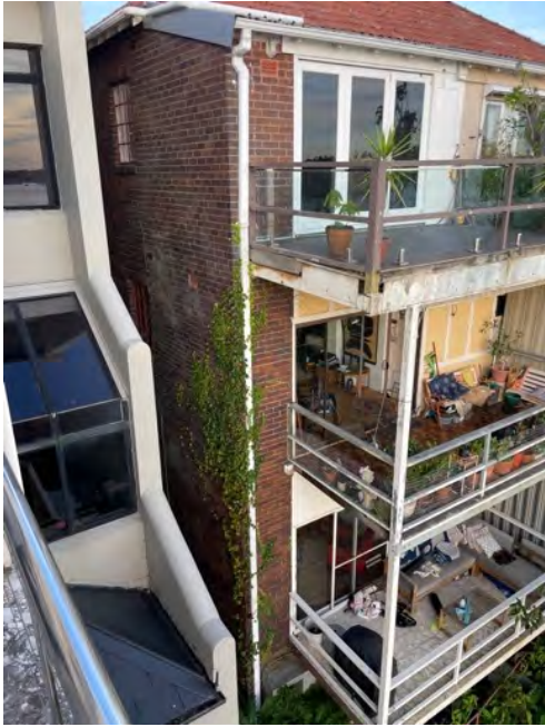
Existing stepped boundary wall, parapet roof and glazing.
