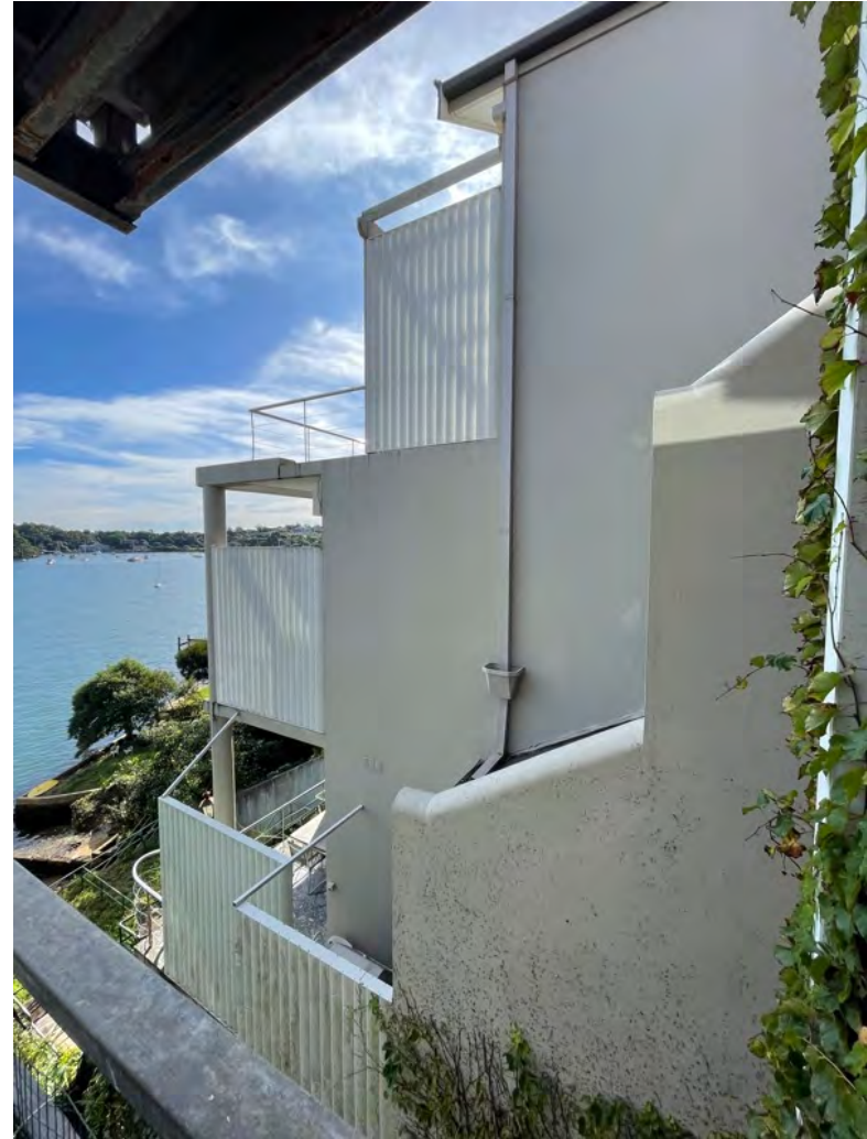
View of existing southern boundary wall from neighbours
