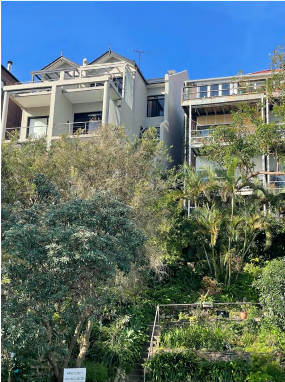
Rear view of existing from waterfront Berrys Bay
