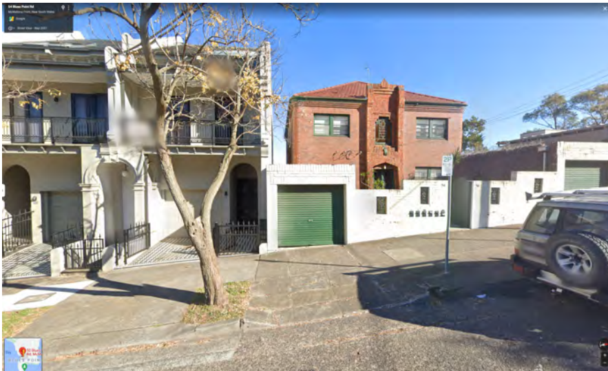
Street view of 54 Blues Point Road
