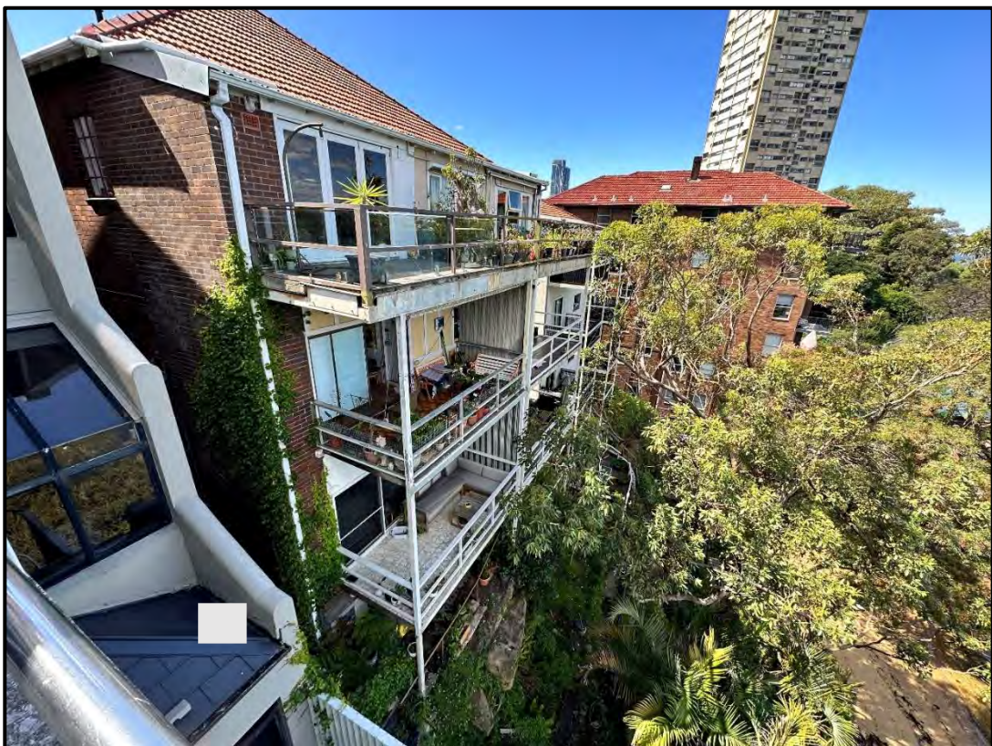
Figure 28: Rear of residential flat building at 46 Blues Point Road
