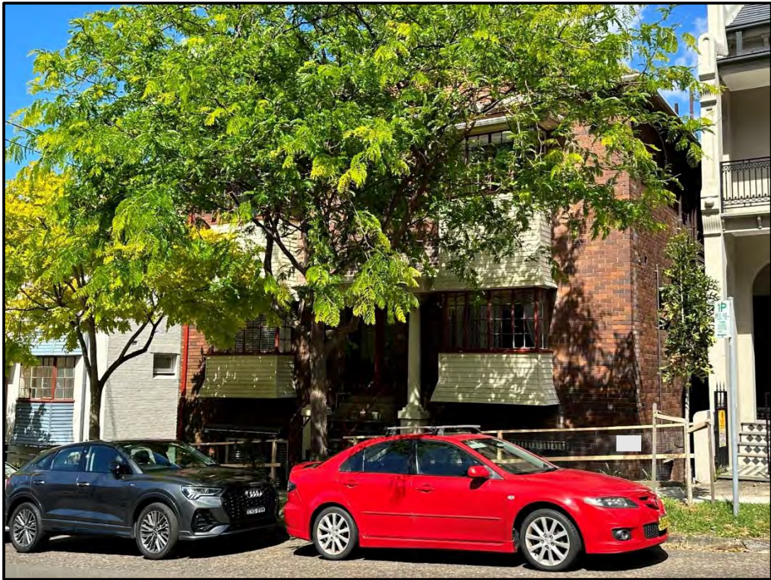
Figure 27: Front of residential flat building at 46 Blues Point Road
