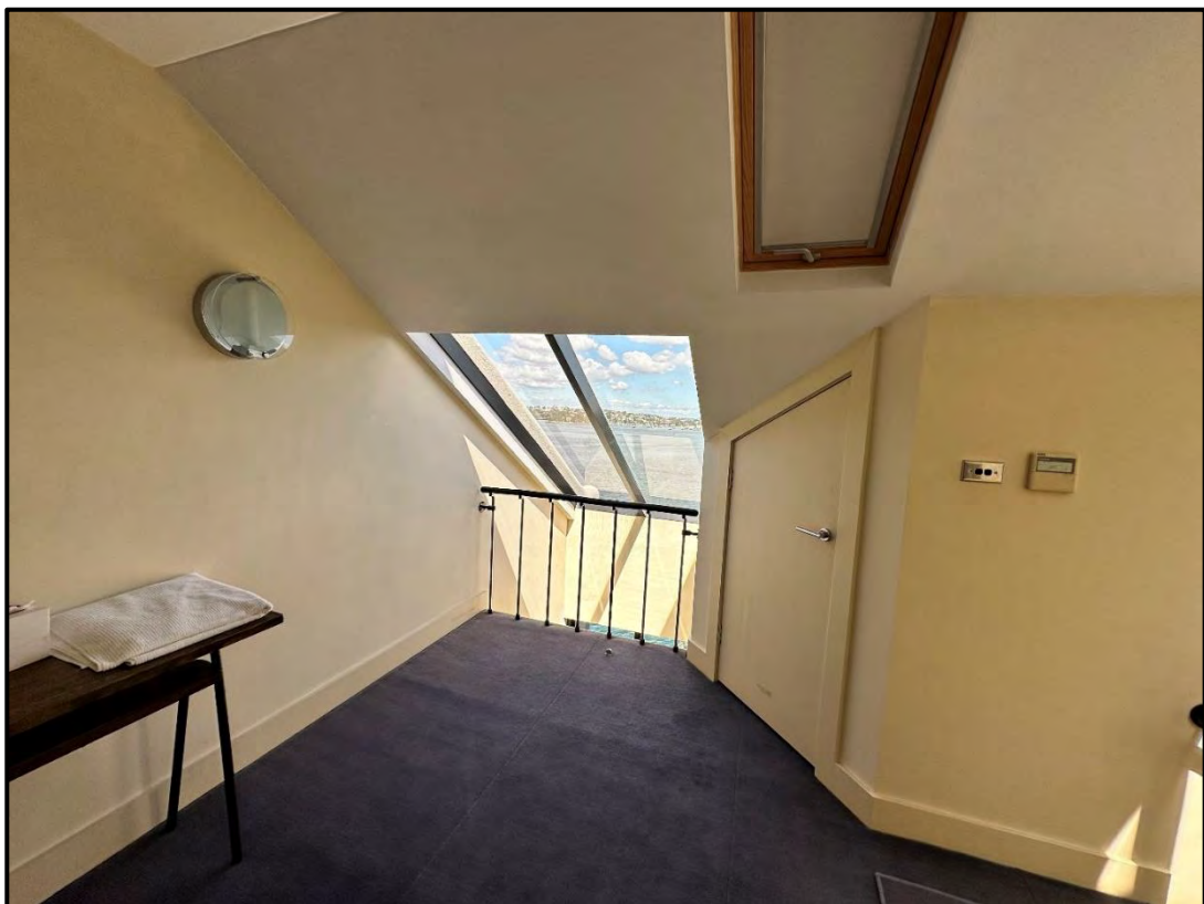
Figure 18: Rear portion of attic level – showing storage room and void
