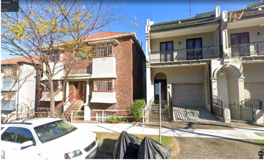
Street view of 46 Blues Point Road
