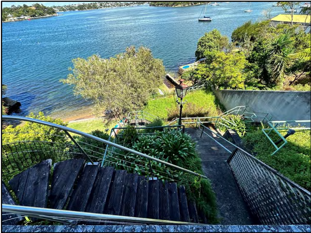
Figure 21: Access stairs leading to rear yard and foreshore area (Berrys Bay) in background
