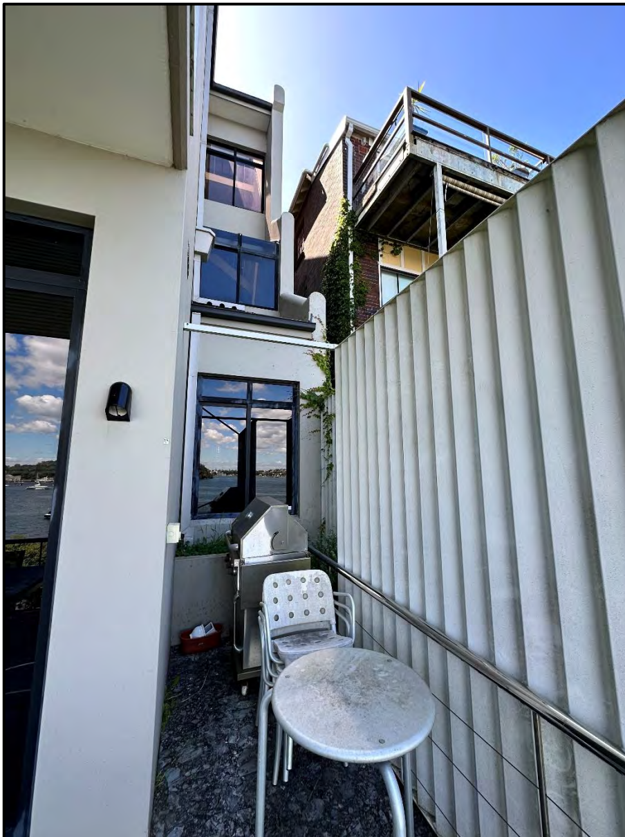
Figure 22: Side setback (southern) of dwelling – taken from lower ground floor
