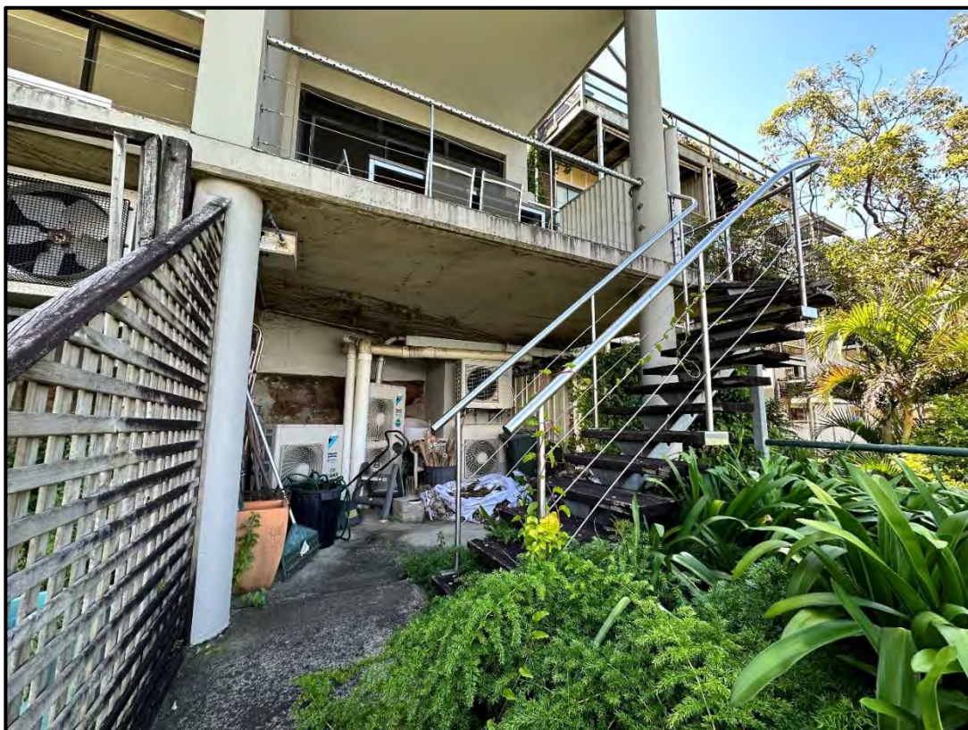
Figure 20: Access stairs leading to rear yard
