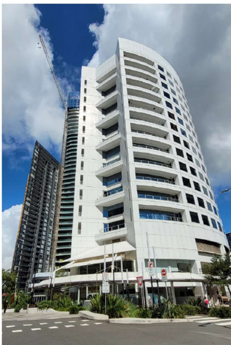
FIGURE 4: View of subject site from corner Atchison Street and Mitchell Plaza, looking south-west.
