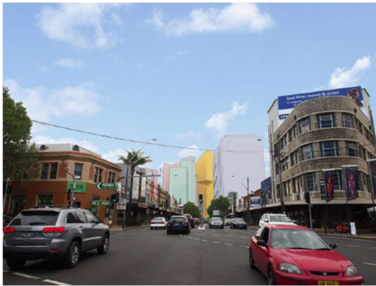
FIGURE 41: Falcon Street, Pacific Highway and Willoughby Road
